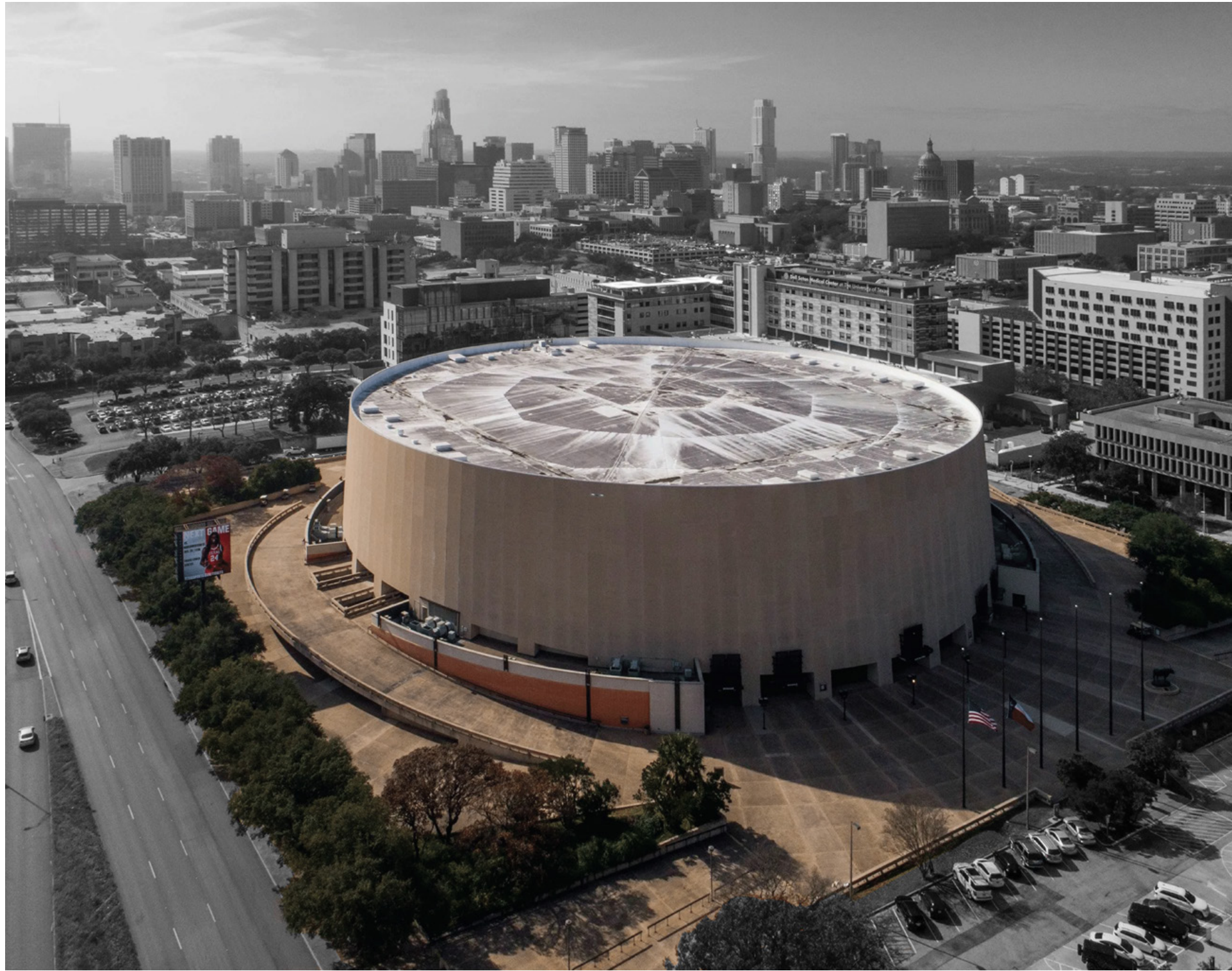
2.01 - Southwest Aerial View of Site
