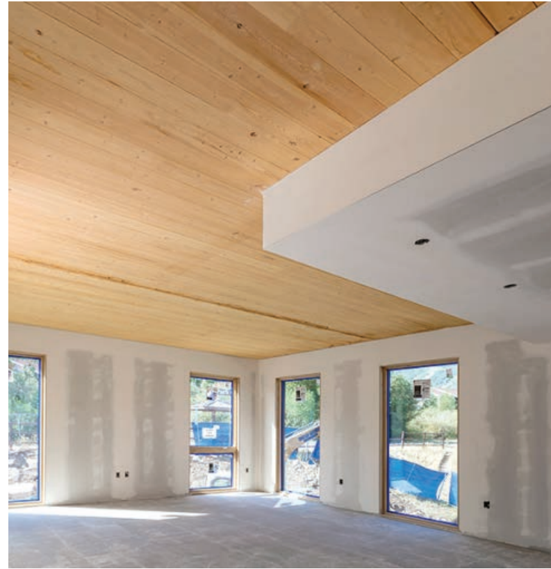
Figure 39: Dry Wall, Exposed CLT and wooden finishes (R&O, 2023)
