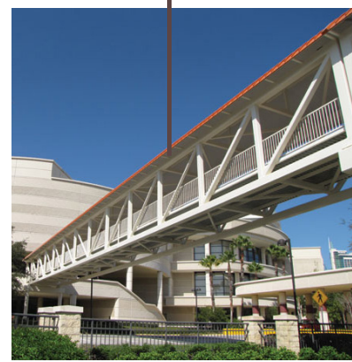
Figure 40 - Warren truss
