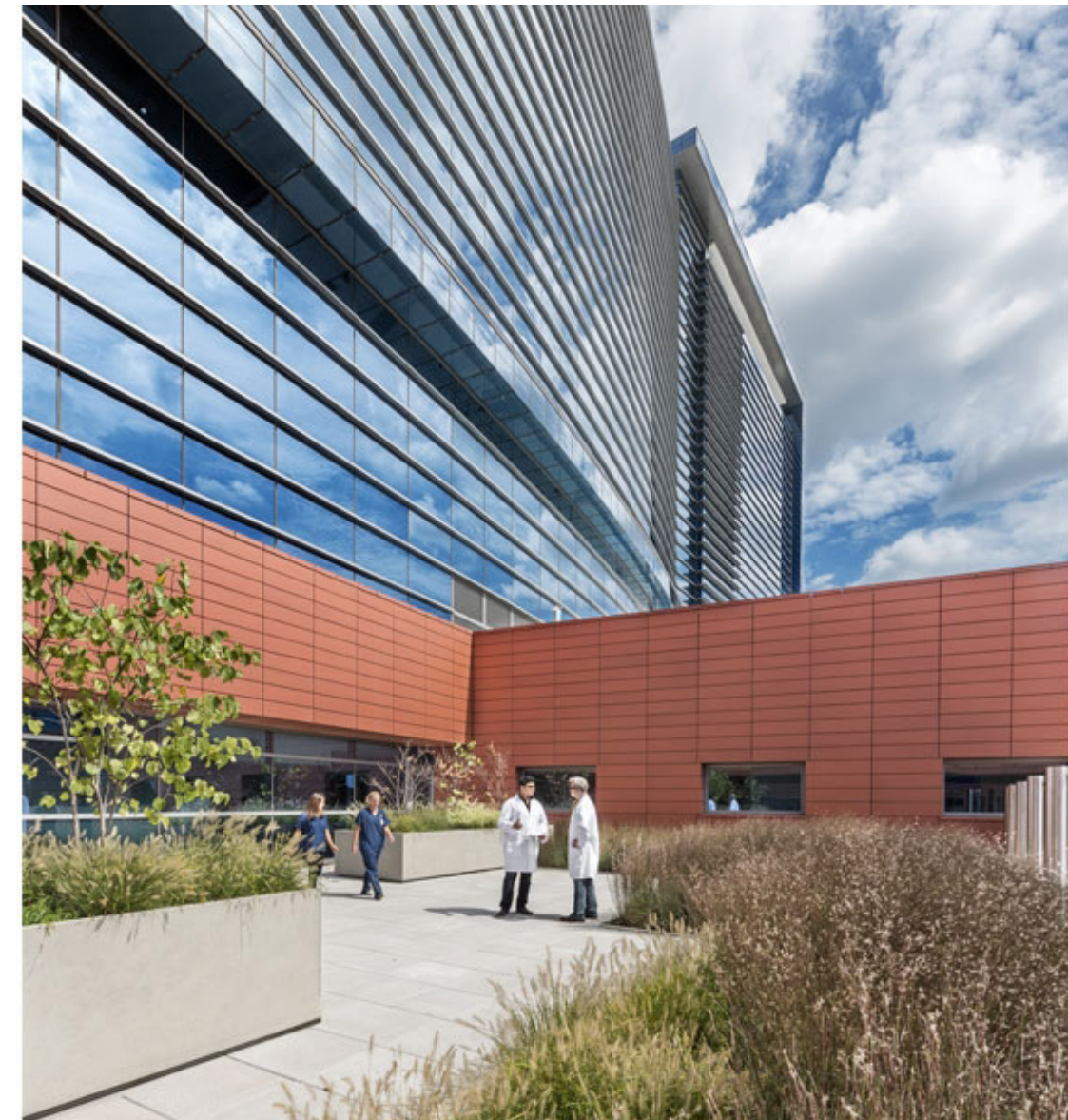
A dedicated roof-top terrace and respite area for staff members offers seating and a place to recharge and relax. ( https://www.eypae.com/client/stamford-hospital/new-stamford-hospital )
