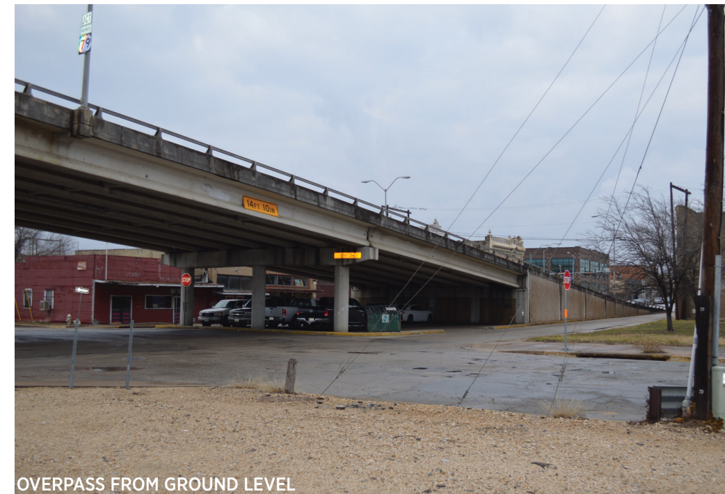
OVERPASS FROM GROUND LEVEL
