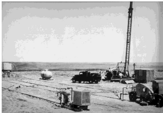
Figure 1.1 First experimental hydraulic fracturing treatment in Grant County, Kansas by Stanolind in 1947 (Smith & Montgomery, 2015).
