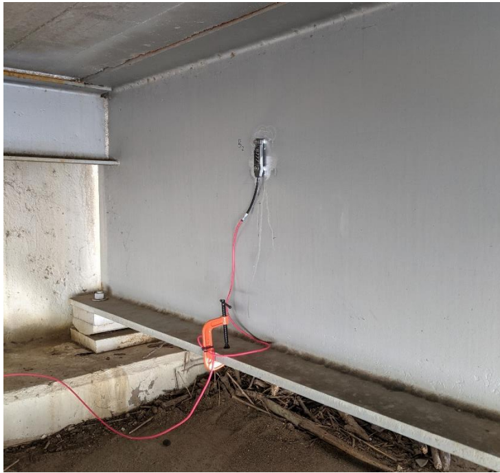
Figure 5.32. Vertical Strain Gauge at North End (Bridge #3).
