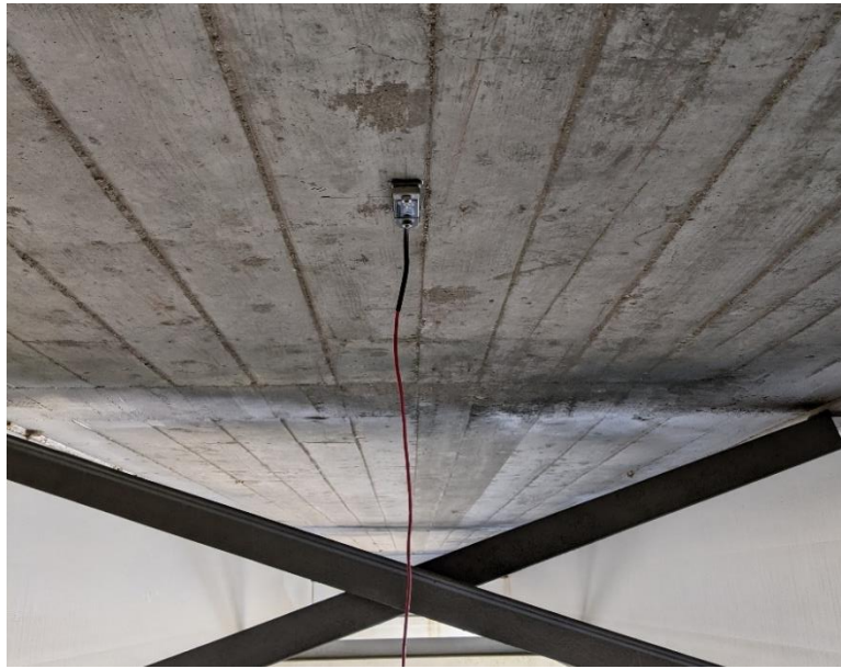
Figure 5.34. Strain Gauge Underneath the Bridge Deck (Bridge #3).
