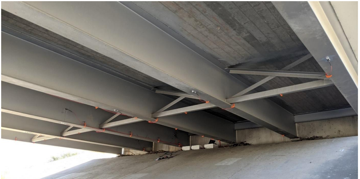
Figure 5.33. Midspan Strain Gauges (Bridge #3).
