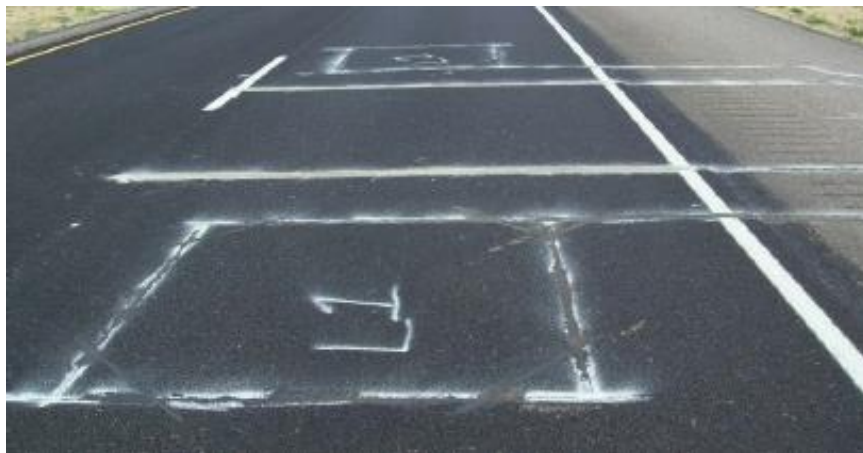
Figure 2.3 Double-Threshold WIM System Setup with Piezoquartz Sensors (reprinted from Hallenbeck and Weinblatt 2004).
