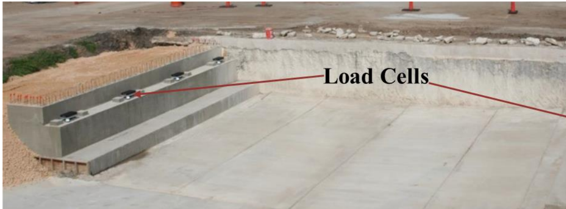
(a) Load Cells at South and North Ends
