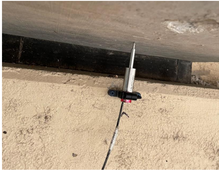
Figure 5.19. LVDT at South End (Bridge #2).
