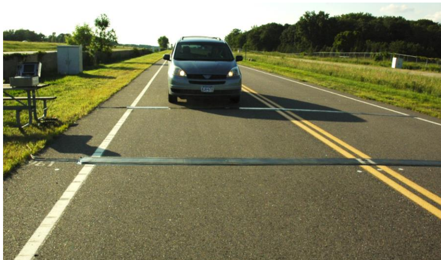
Figure 2.6. Installed Weigh Pads with Air Cavity and the Test Vehicle (reprinted from Kwon 2012).
