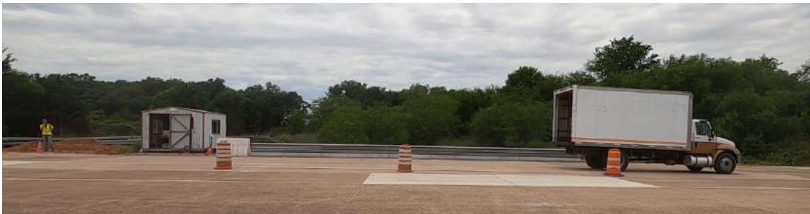
(c) Vehicle Left the RELLIS Bridge
