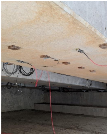
(c) Strain Gauges Installed at Midspan
