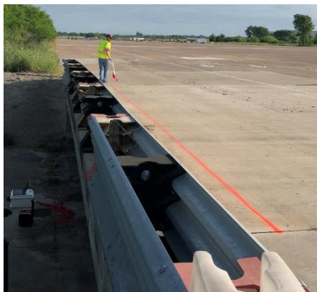
(b) Spray Paint to Mark the Lanes
