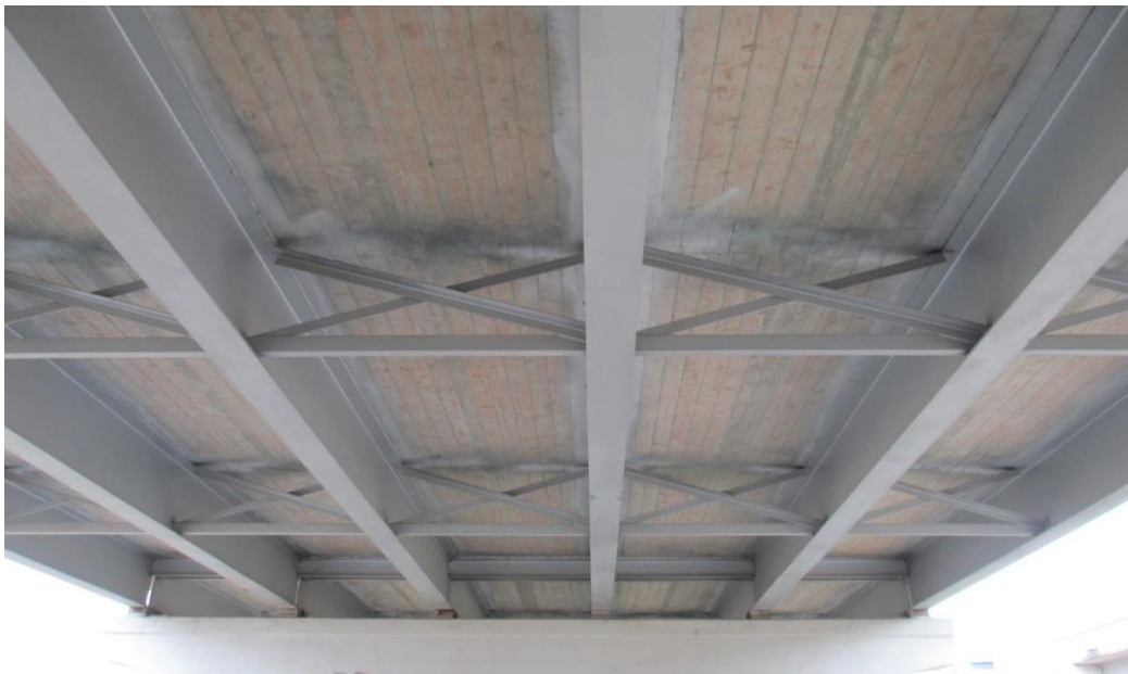
Figure 4.9. Bridge #3 Underside View.
