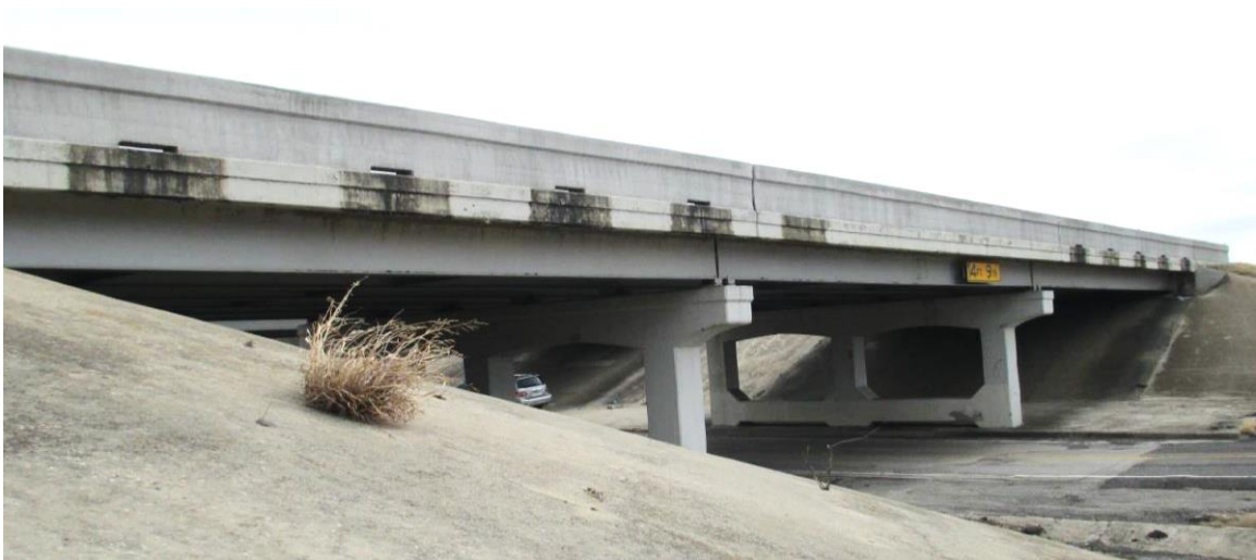
Figure 4.8. Bridge #3 Elevation View.
