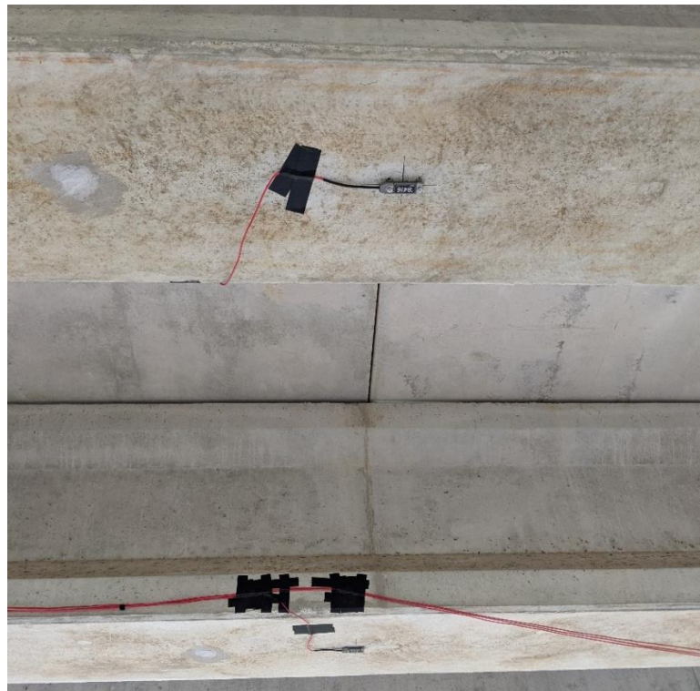
Figure 5.20. Midspan Strain Gauges (Bridge #2).
