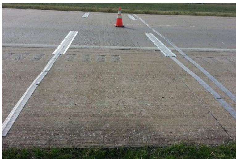
Figure 2.8. Two-Lane Portable WIM System Deployment (reprinted from Refai et al. 2014).
