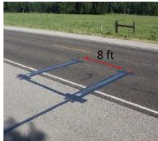
(b) Piezo Sensor Installation Using Custom-Devised Metal Plates
