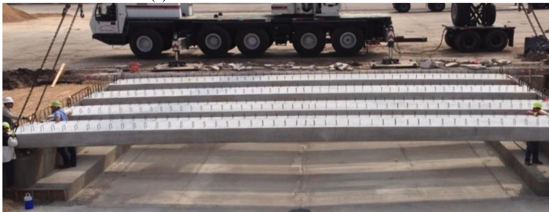
(b) Slab Beam Placement
