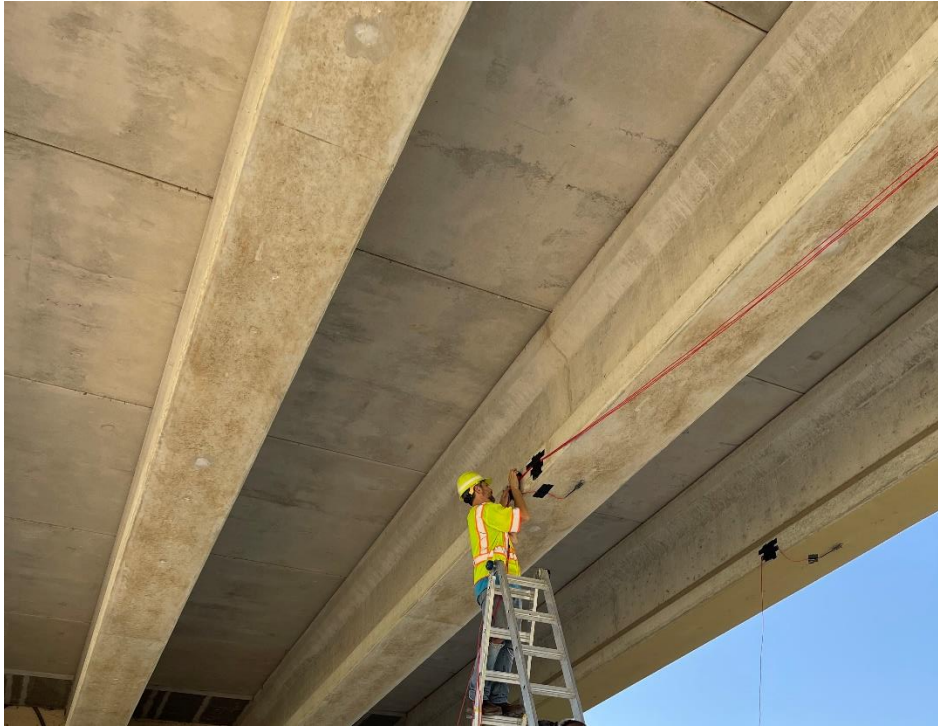
Figure 5.21. Installing Strain Gauges (Bridge #2).
