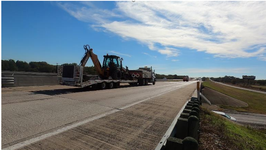
Figure 5.41. Truck B Passing the Inside Lane (Bridge #3).
