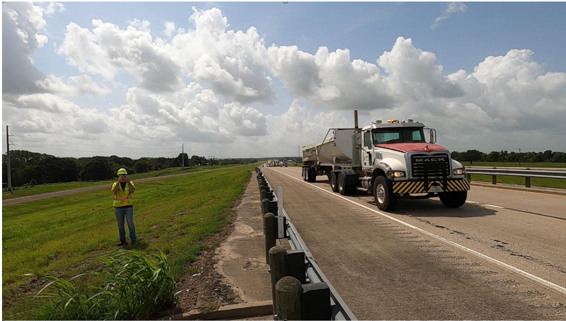
Figure 5.25. Truck Passing the Outside Lane (Bridge #2).
