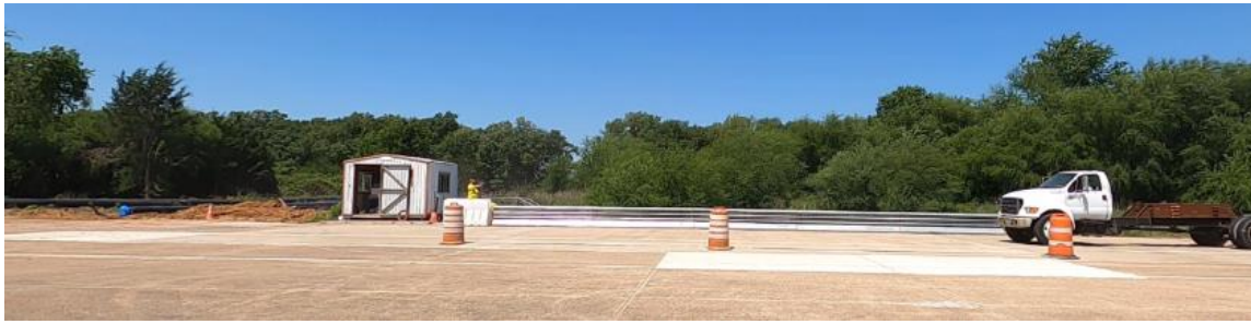
(a) Vehicle Entered the RELLIS Bridge from the North
