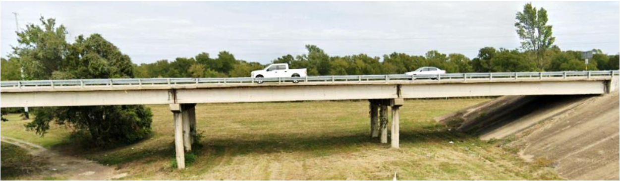
Figure 4.3. Bridge #1 Elevation View.
