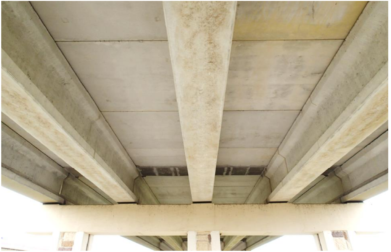
Figure 4.6. Bridge #2 Underside View.
