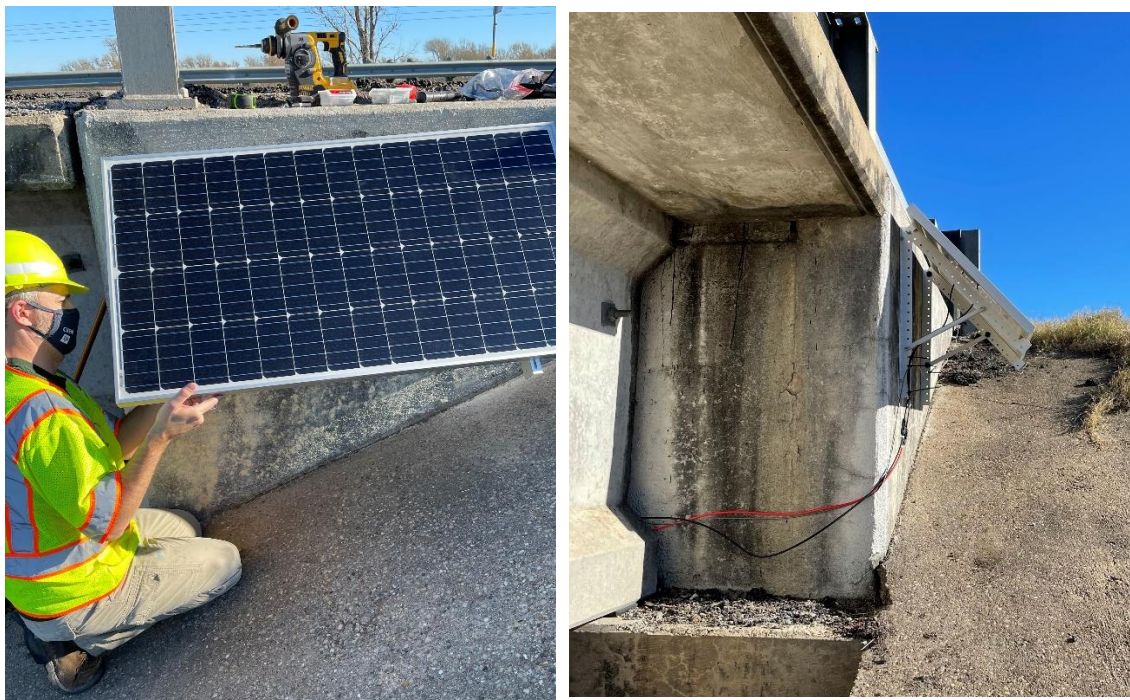
Figure 5.7. Installation of the Solar Panel.
