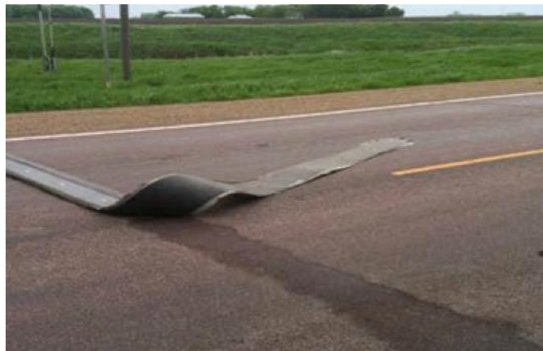
Figure 2.7. Weather-Pulled Pads (reprinted from Petersen et al. 2015).
