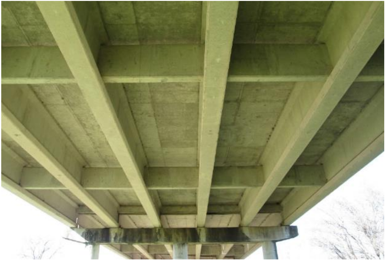
Figure 4.4. Bridge #1 Underside View.
