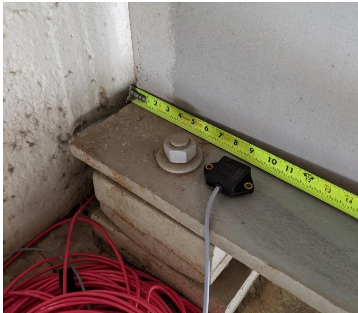
Figure 5.31. Accelerometer at North End (Bridge #3).
