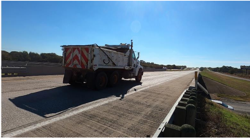
Figure 5.40. Truck A Passing the Outside Lane (Bridge #3).
