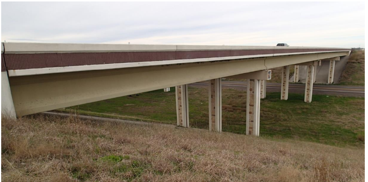
Figure 4.5. Bridge #2 Elevation View.
