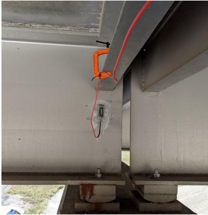
Figure 5.30. Vertical Strain Gauge at Second Span (Bridge #3).
