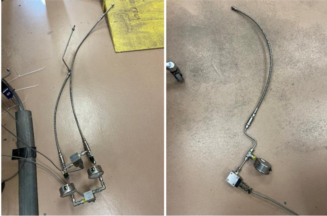
Figure 60. Change from hard lines to flex lines to reduce connection wear.
