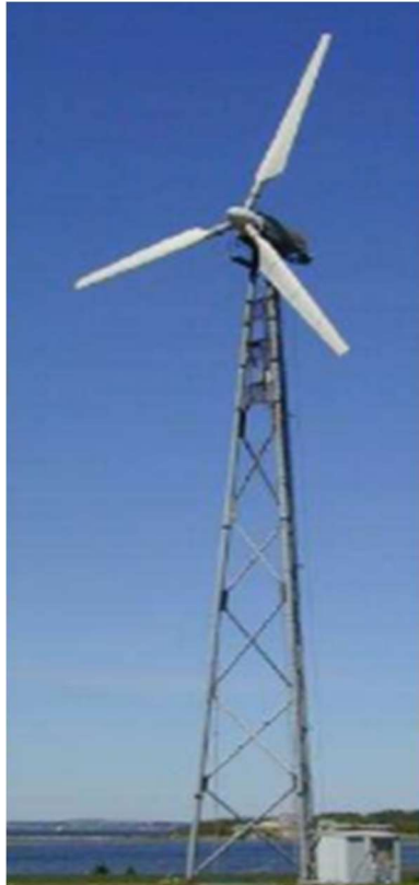
Figure 5-1: Lattice-type wind turbine tower (DNV/Risø, 2002)
