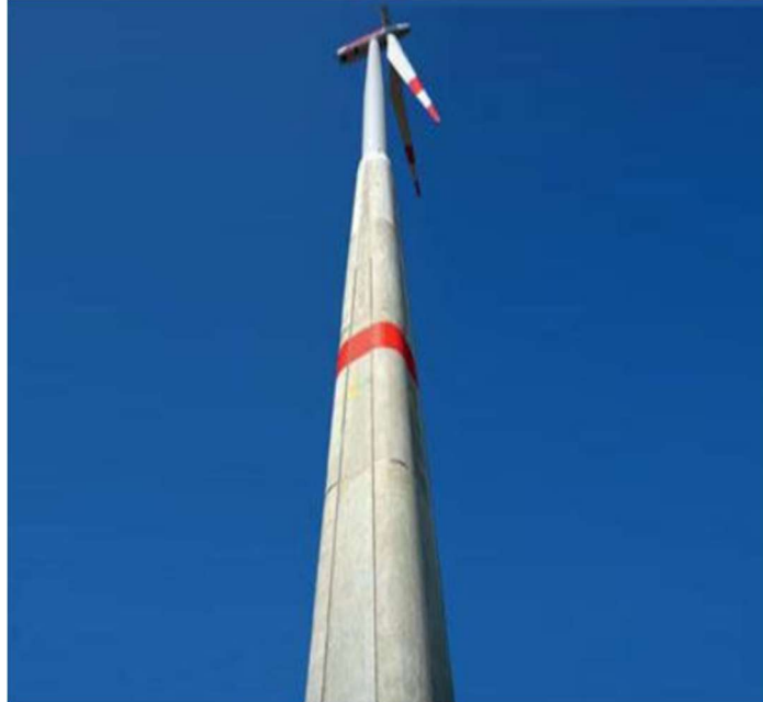
Figure 5-4: Example of hybrid tower (Anonym)
