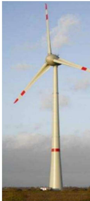
Figure 5-3: Tubular Reinforced Concrete Towers (DNV/Risø, 2002)
