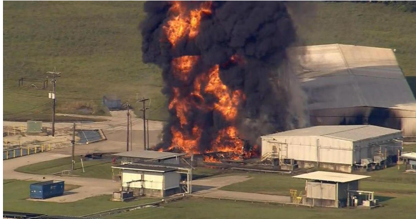
Figure 14: Arkema chemical plant fire (Reprinted from [22]. CBS News, 2017.)
