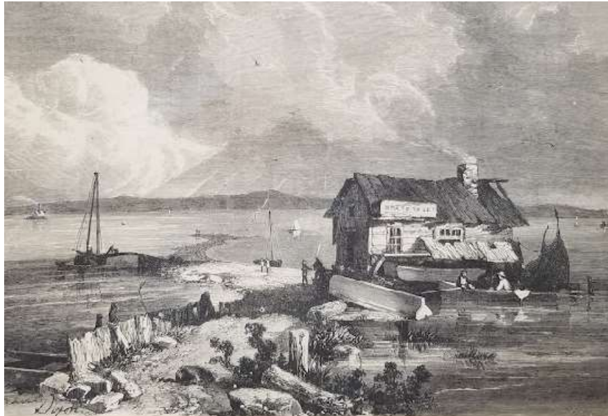
In 1812 William J. Vredenburg, one of the earliest influential residents, hired the shipwright Charles Burnett to construct a yacht for him to entertain guests. This yacht was completed in 1816 and named The Four Sisters . It had a length of 42 feet (12.8 meters) and a beam 10 feet (3.0 meters). 121 This was the first of many yachts to come. Figure 16: A mid-19th century sketch of Skaneateles Lake showing a boat rental house with rowboats and sailing boats by J.P. Dixon (Skaneateles Historical Society).
