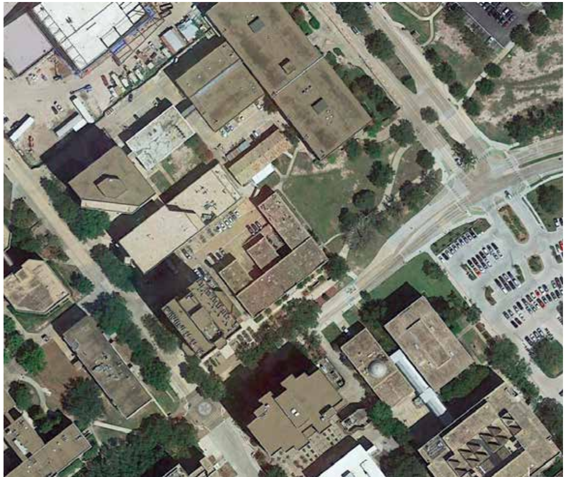
Figure 2: Aerial view of Haynes Engineering Building. Google Earth.
