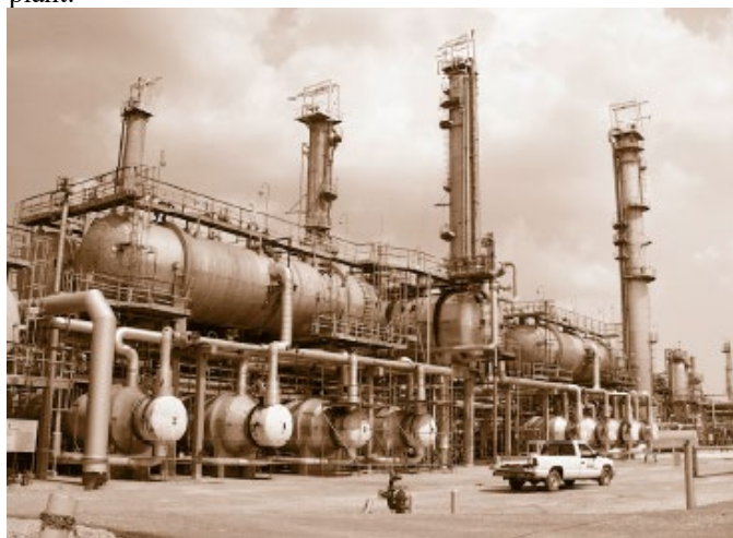
Figure 49: Alkylation Plant (Courtesy of Motiva)
