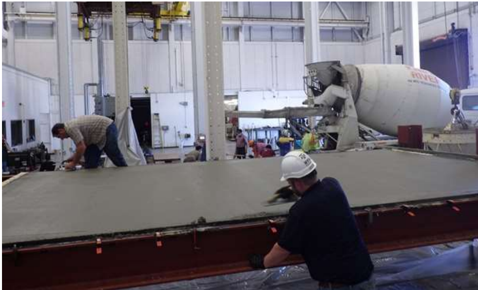
Figure 74: Slab finishing (image by Matthew Yarnold)
