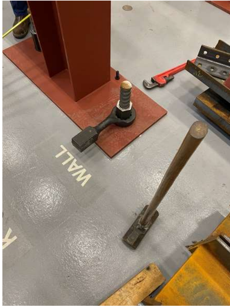
Figure 45: Stub column connection to CIR strong floor with tension rods
