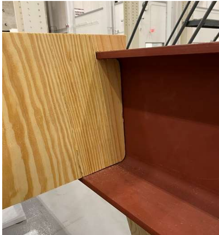
Figure 64: Floor system concrete plywood end form, beam scribed
