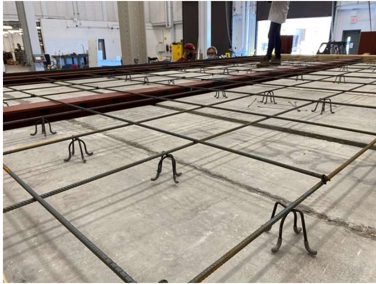
Figure 69: Concrete slab rebar reinforcement tied mat, close up
