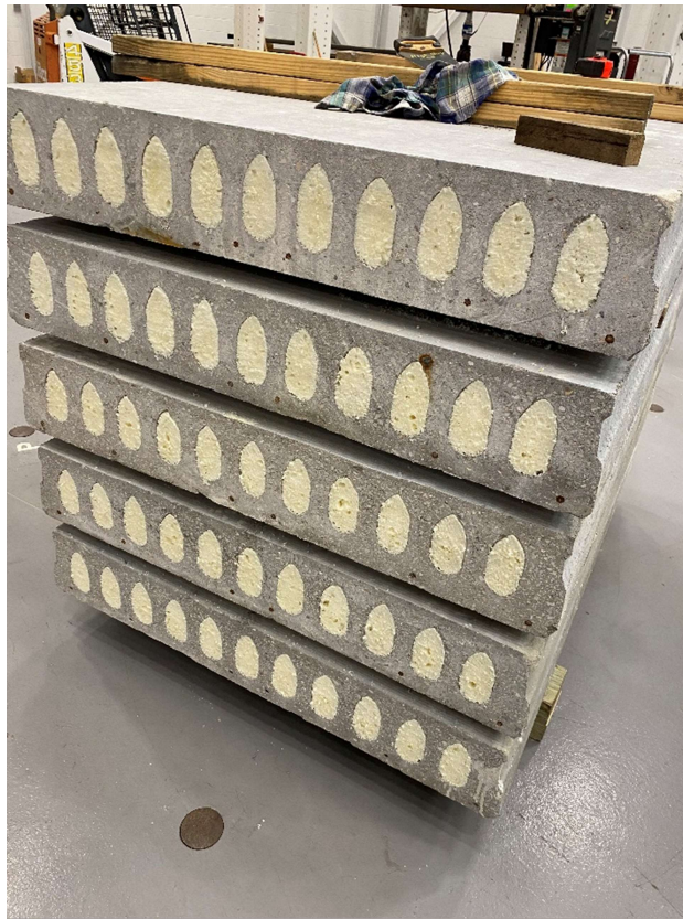
Figure 61: Pre-cast hollow-core concrete panel foam closure after cutting
