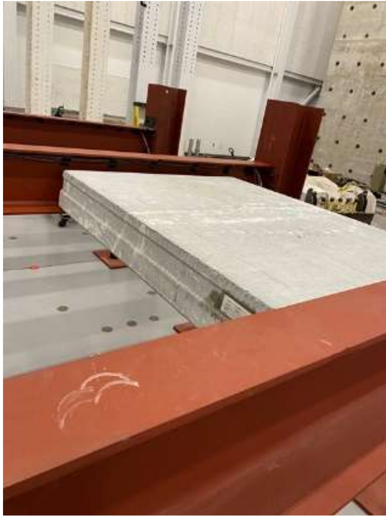
Figure 57: Construction loading of the steel frame – first concrete pre-cast panel
