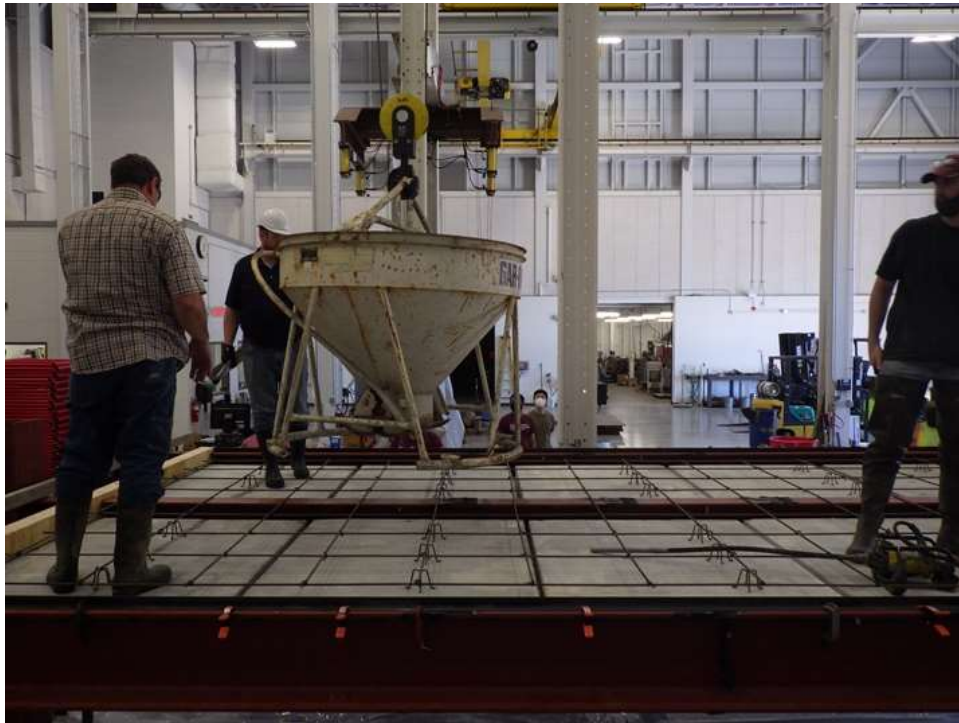
Figure 71: Slab pour, concrete dump bucket (image by CIR Staff)
