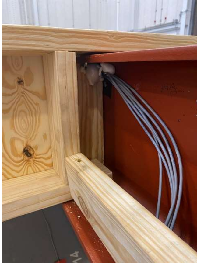
Figure 67: Concrete form wire sealing
