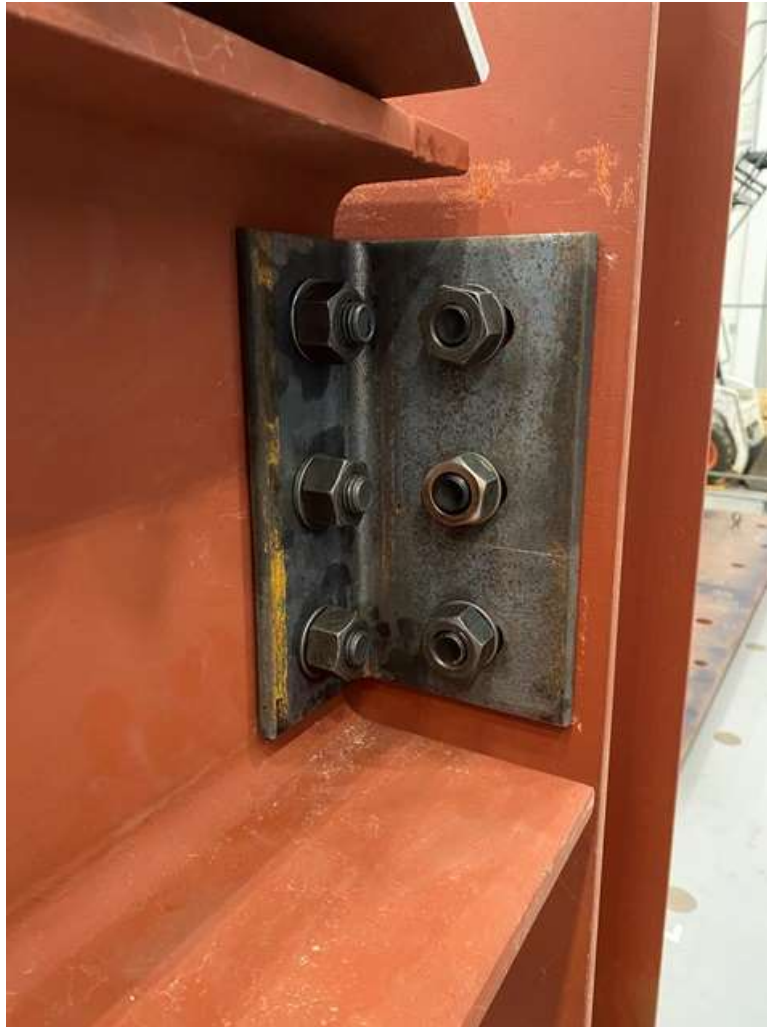
Figure 38: Beam to column shear connection with slotted holes, installed
