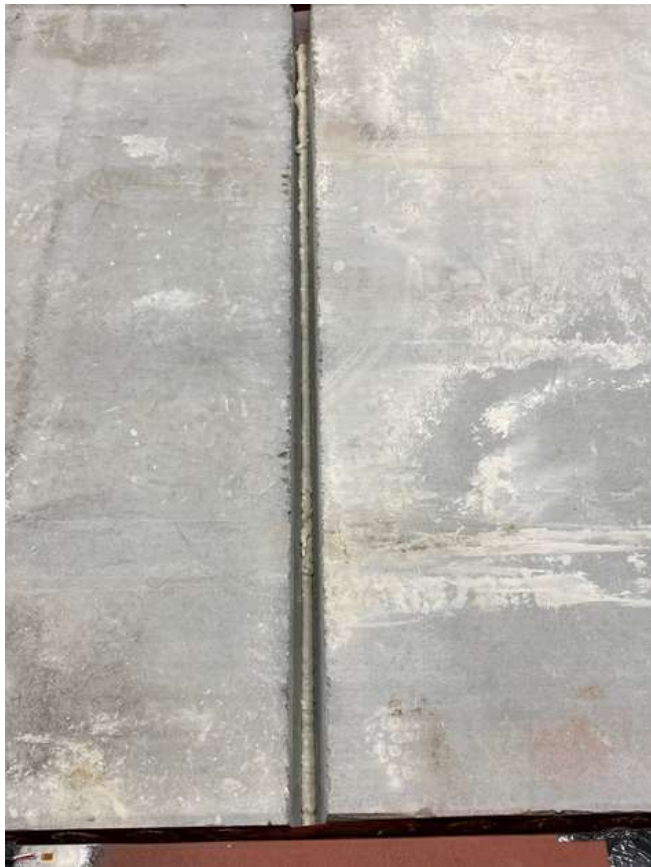
Figure 62: Joint sealing between pre-cast concrete panels
