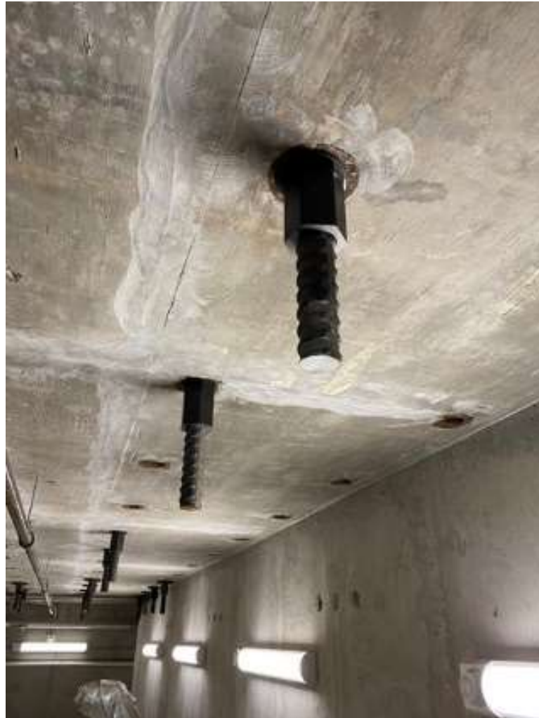
Figure 44: CIR tension rods basement connection
