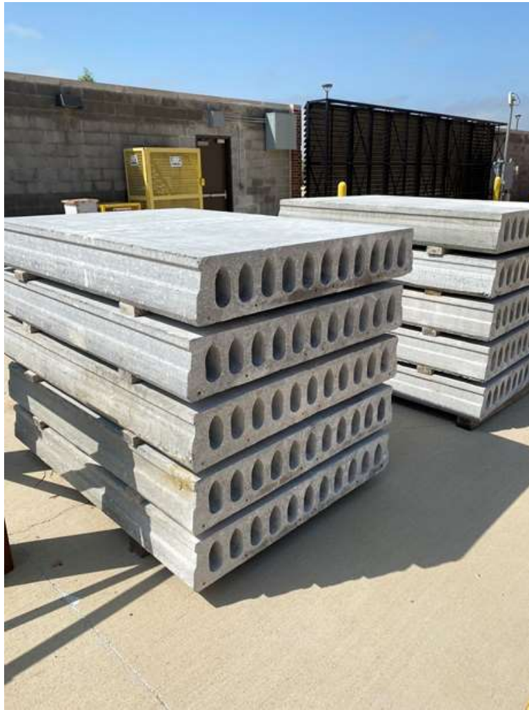
Figure 54: Pre-cast hollow core concrete panels
