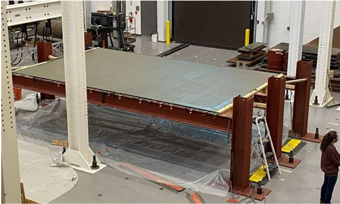
Figure 75: Finished concrete slab
