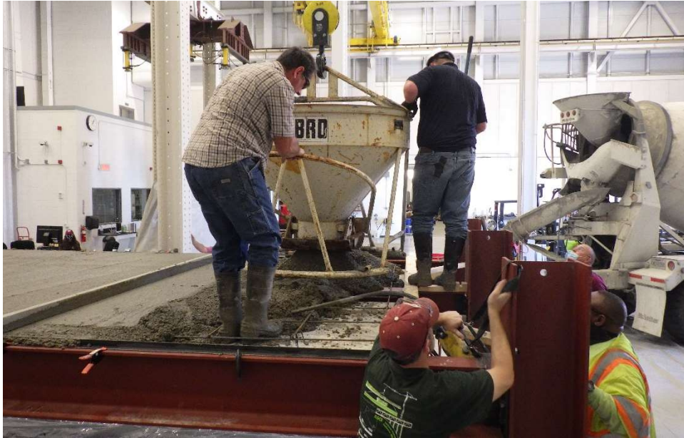
Figure 73: Slab pour and screeding surface (image by CIR Staff)
