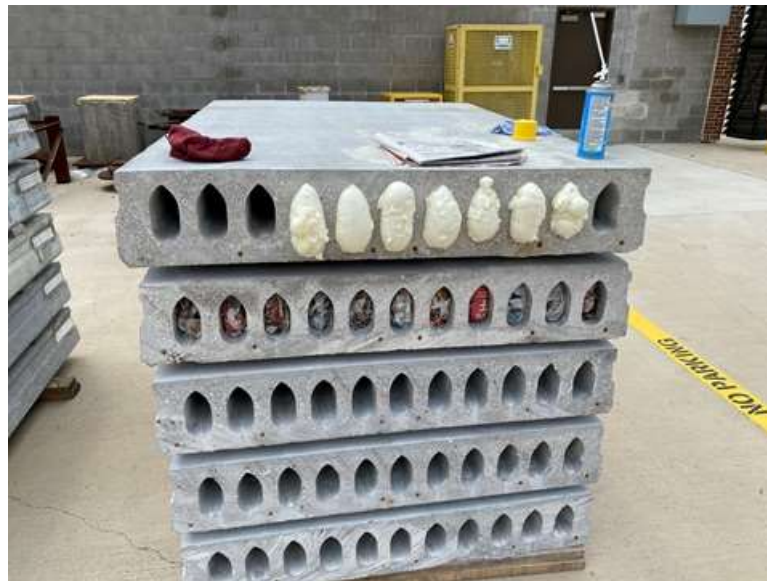
Figure 60: Pre-cast hollow-core concrete panel foam closure
