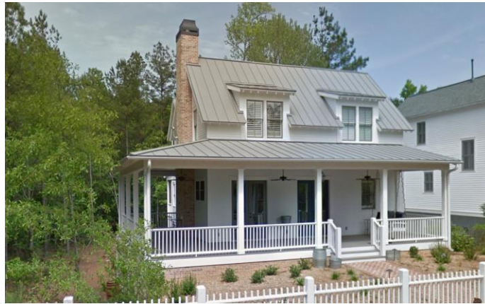
Figure 4.6: Building C in the Serenbe Community. Source: Modified from Google Map 2021.
