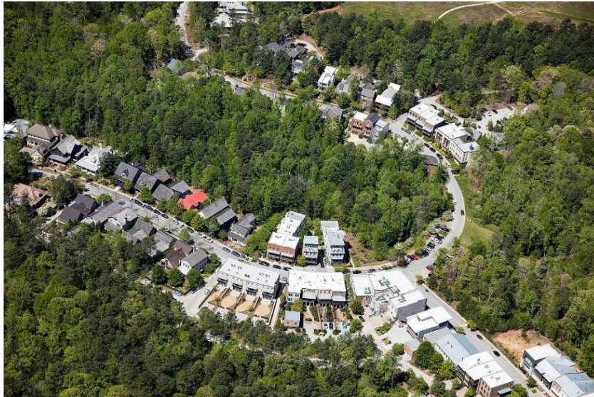
Figure 4.2: Aerial view of Selborne hamlet in the Serenbe community. Source: Serenbe Development.
