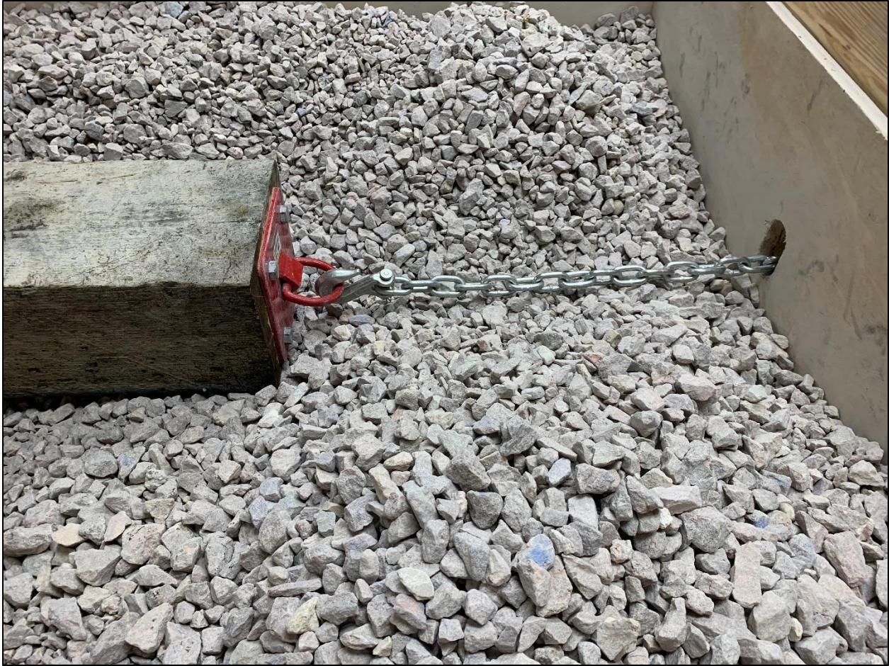
Figure 14: Checking for correct crosstie height and alignment
