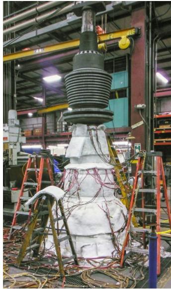
Figure 5: Example setup for a post weld heat treatment [10].
