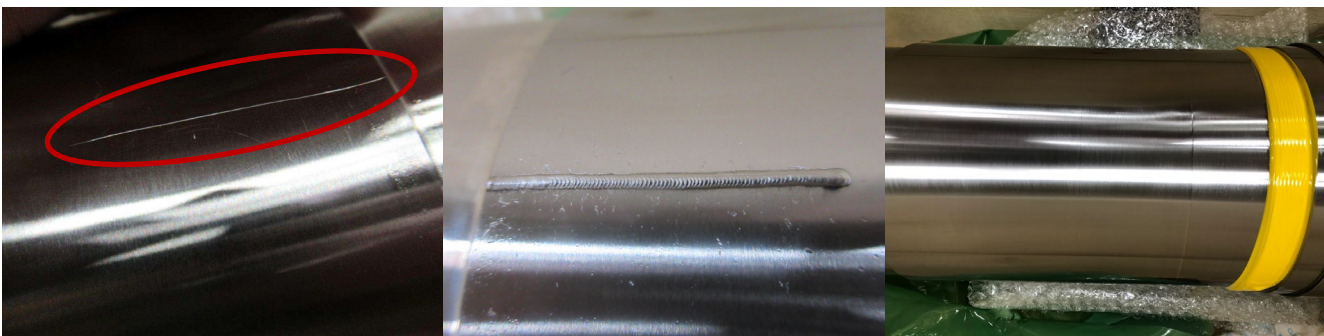
Figure 9: The scratch, which has been circled, in a journal area (left), the same scratch after LBW repair (middle), and the repaired area after final machining (right).
