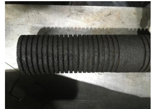
Iron sulphide sludge observed on upstream cartridge filters
