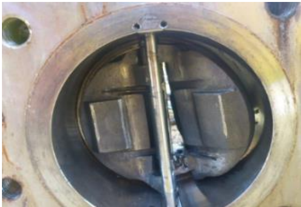
Check valves at 2 nd , 3 rd & 4 th stage found parted and/or passing
