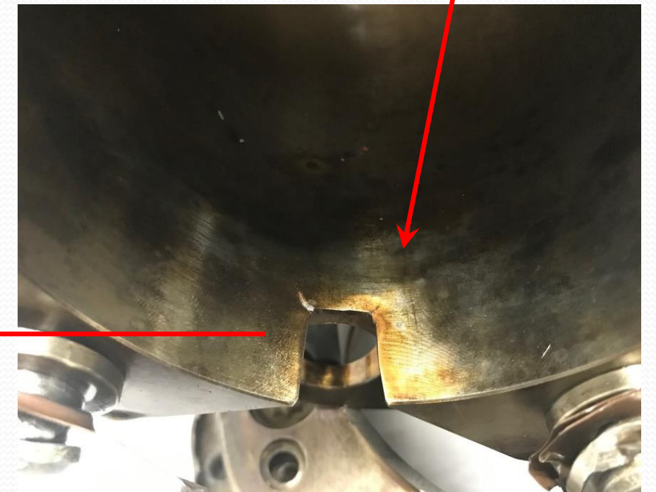
Findings are similar for First failure and Second failure
