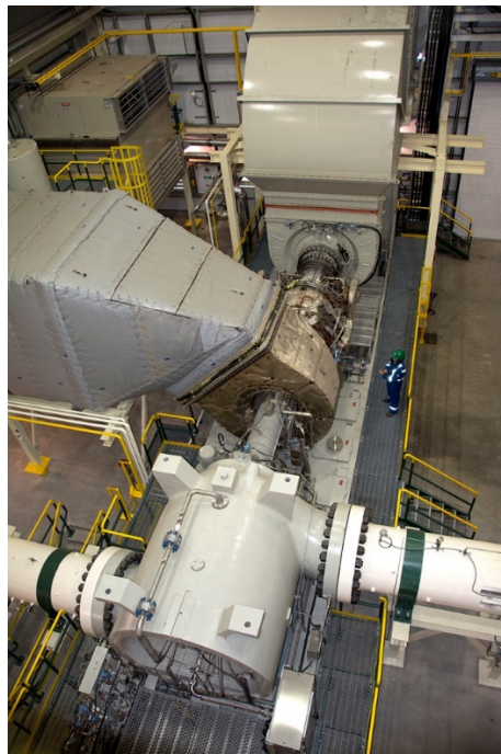
Figure 1: Industrial Gas Turbine powers a gas compressor
