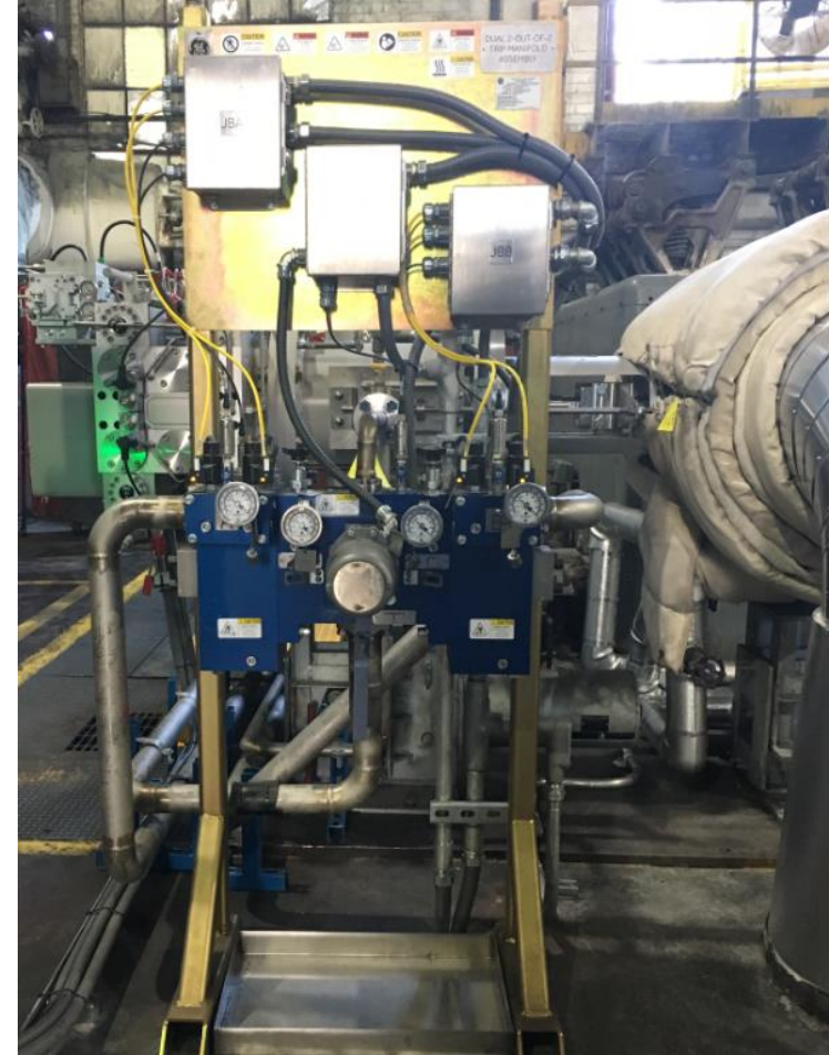
TMA mounted with T&TV in background
