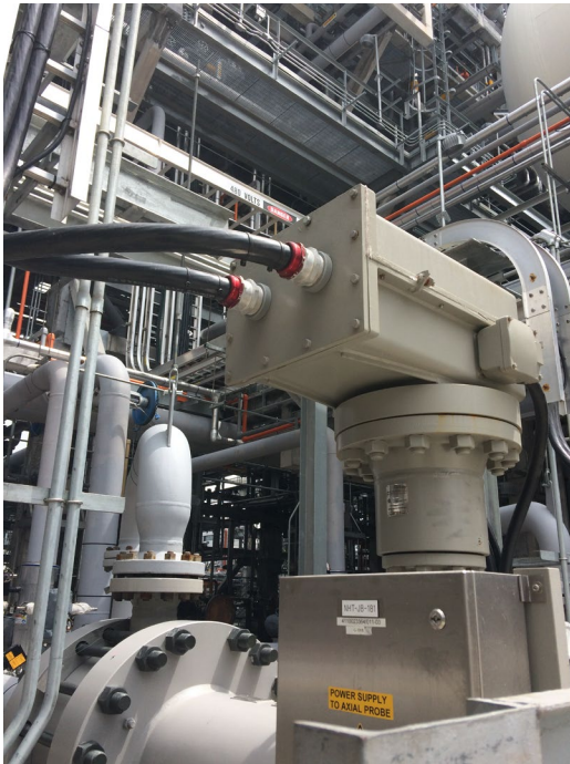
Figure 7 Oversized electrical boxes to accommodate larger wires
