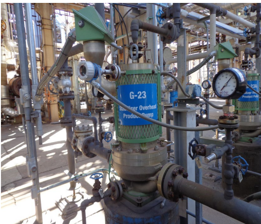
Figure 6 Vertical canned motor pumps to reduced radial load of rotor
