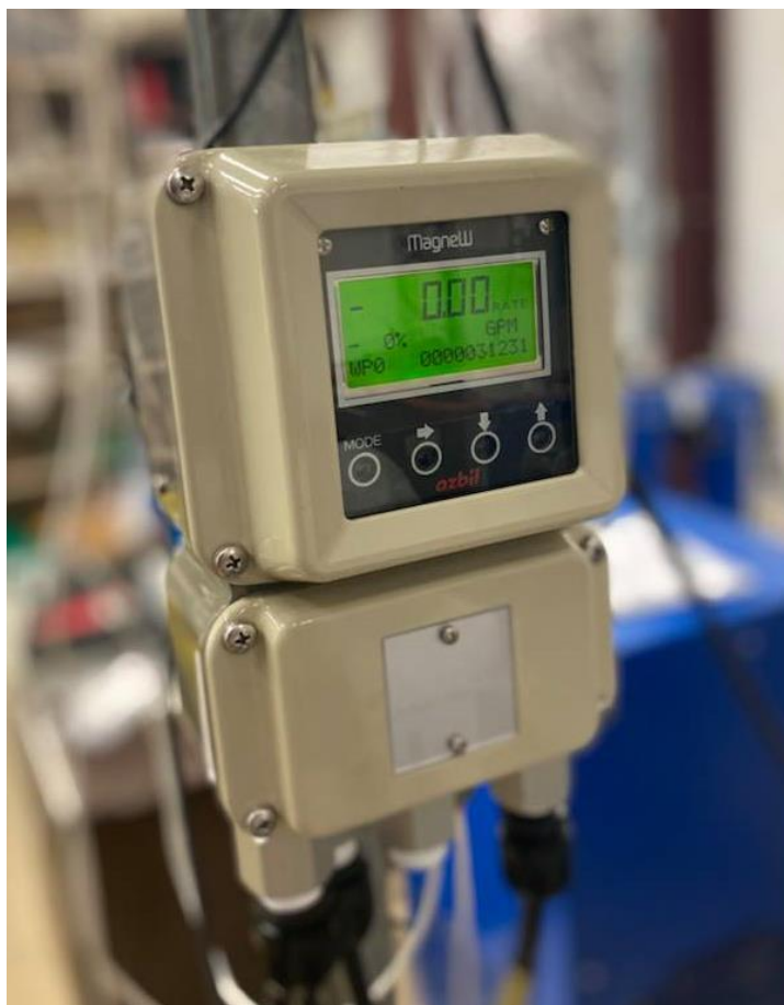
Figure 3.23 Magnetic Flowmeter converter at the water injection line. The converter of a product number (MGG14C-MH4H-1B1N-YAH) and serial number (R-F3396-A1-011)
