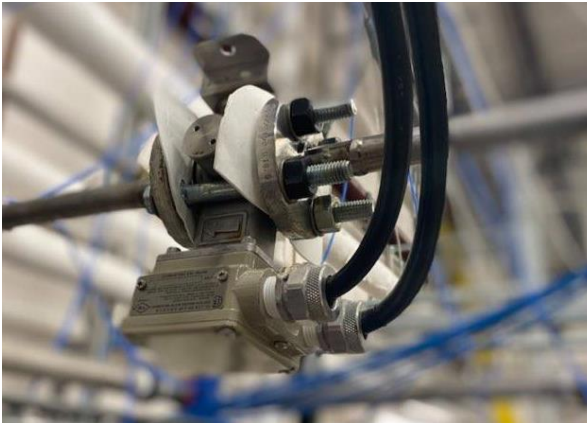
Figure 3.22 Magnetic Flowmeter detector at the water injection line. The detector has a model number of (MGG18D-015P21LS5AAA-XX-Y) and a product number of (R-9AH1E-41-021A).
