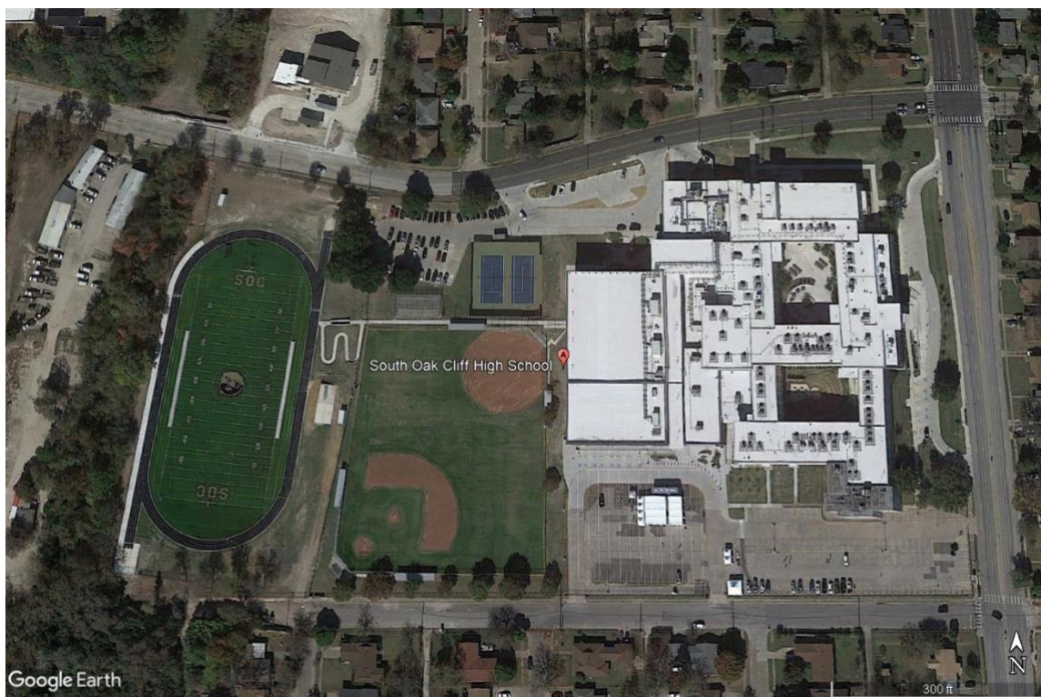
Figure 2.1 South Oak Cliff High School Campus. Source: Google Earth
