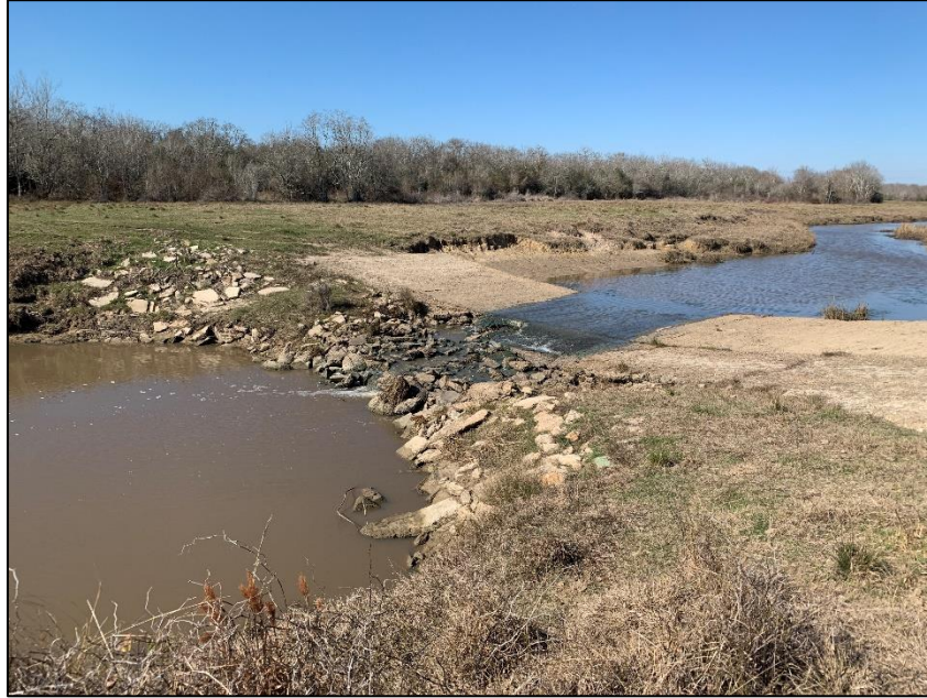
Figure 16. Barrier to flow on Big Boggy Creek. This structure (barrier 1 in Table 2 & Figure 15) does not appear to have culverts and instead allows the water to flow over the top.
