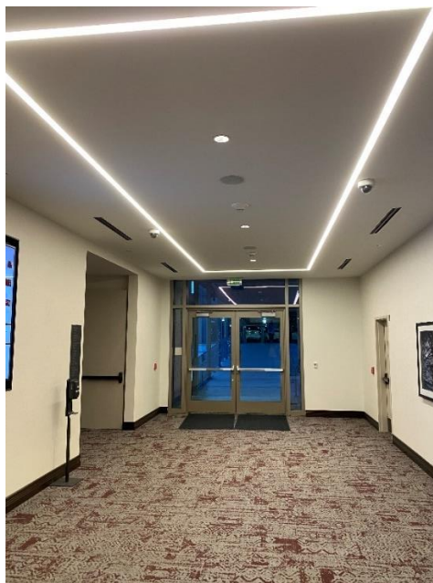
Figure 5.32: LEDs in the common passage of Texas A&M Hotel
