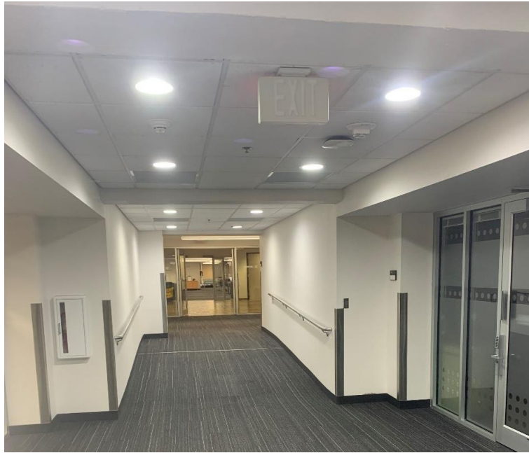
Figure 5.19: LED lighting on second floor: 5 ft. height
