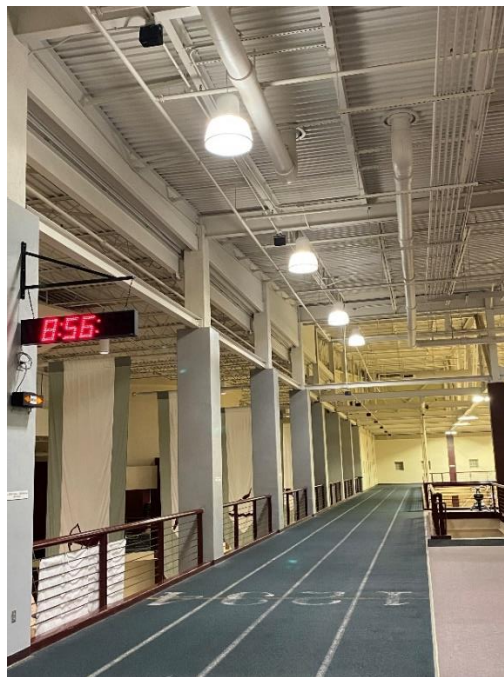
Figure 5.39: High Bay LEDs on running track (at 12 ft. distance)
