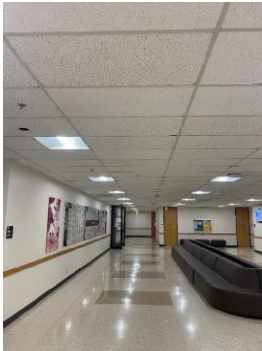
Figure 5.16: LED lights (5 ft. height)
