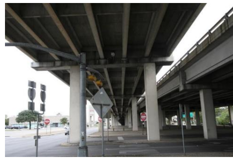
(b) Double column bent
