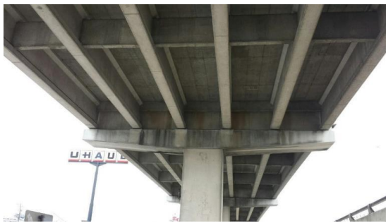
(a) Single column bent
