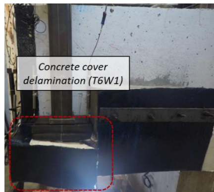
(c) Concrete cover delamination
