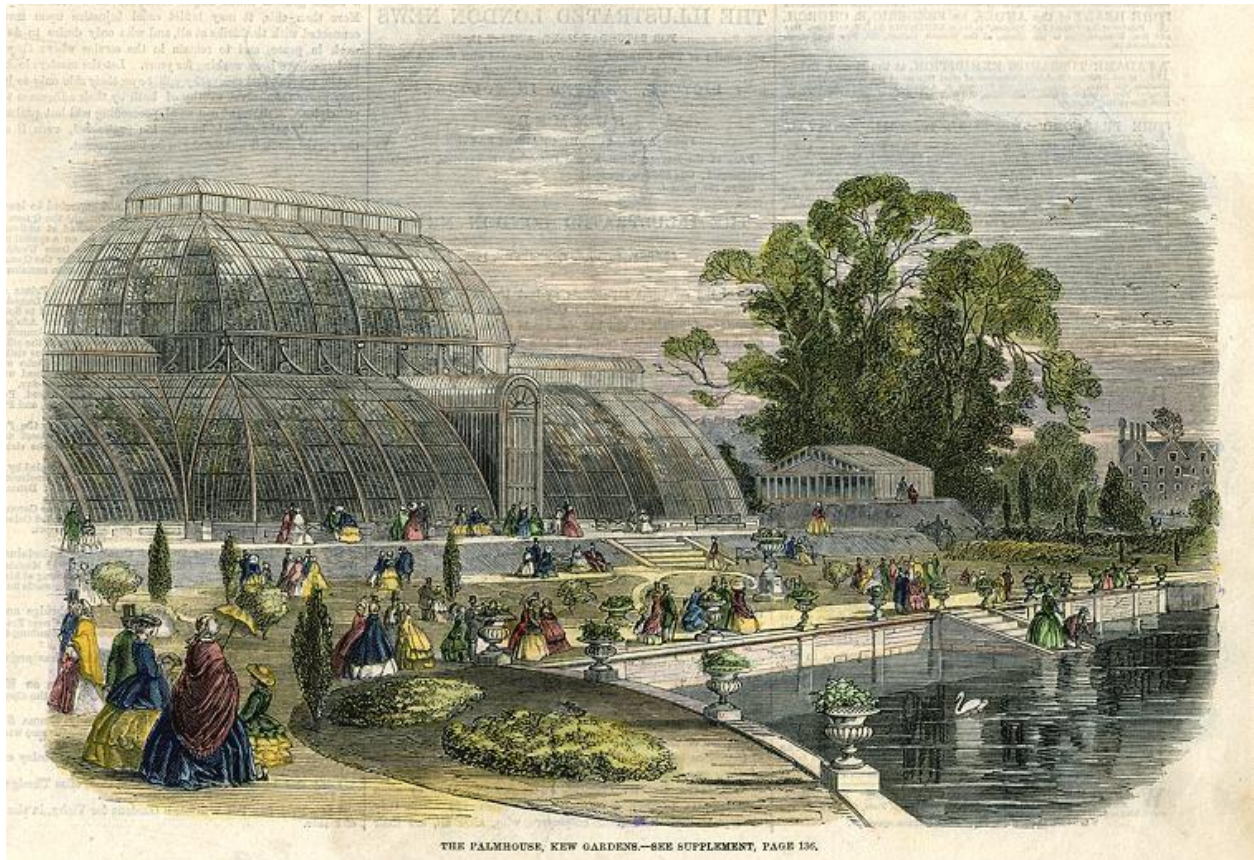
Fig. 3.3 The Palm House, Kew Gardens. Published in The Illustrated London News , Aug. 1859. Wood engraving with hand colour.
