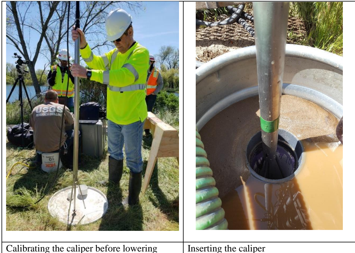
Figure 26. Caliper calibration and installation in the borehole
