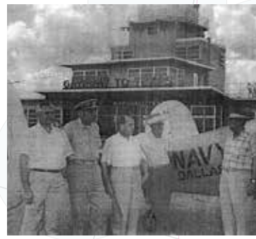
Unknown Gentlemen Posing in Front of the Terminal. The "Gateway to Texas" sign was added after construction and removed at some point. This image was taken in the early 1950's (6)
