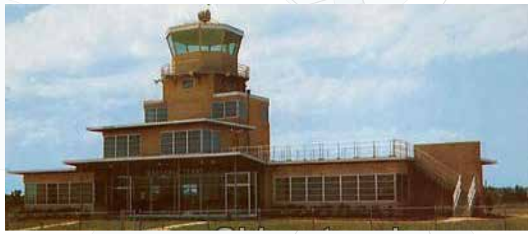
Airside view of the Harrison County Memorial Airport Terminal (7)
