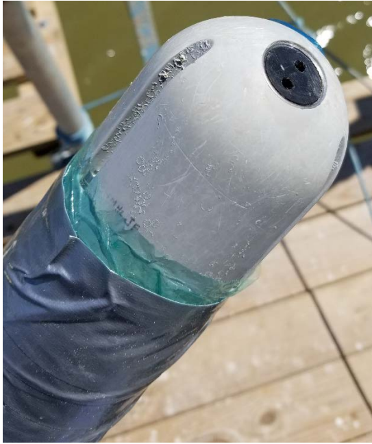
Fig. 12 – Photograph of the ADCP pressure transducer (round black section)
