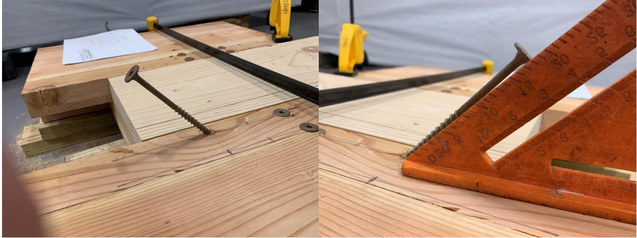
(a) (b) Figure 3.12. 45 Degree Fastener Installation
