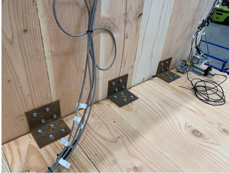
Figure 6.42. Test B3 Wall-to-Floor Connections After Testing
