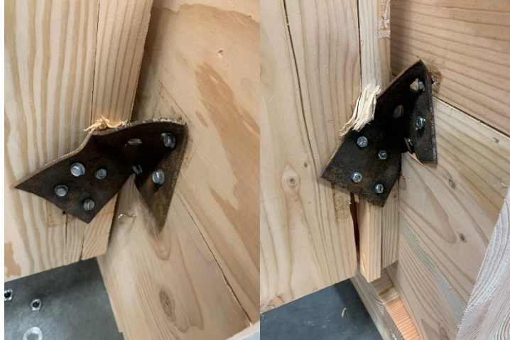
Figure 3.37. Non-Load-Bearing Wall-to-Floor Monotonic Test Failure
