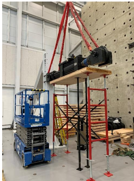
Figure 6.19. Shoring Used to Support Actuator
