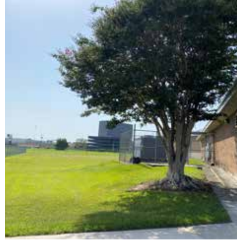
SOUTH VIEW OF WALL & MECHANICAL SYSTEM
