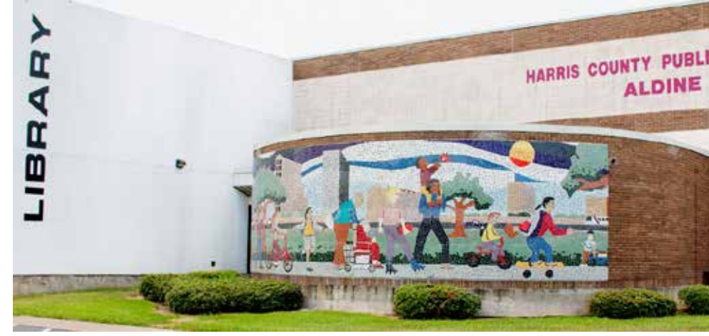
AFTER 2001 RENOVATION- NORTH EASTERN VIEW OF LIBRARY
