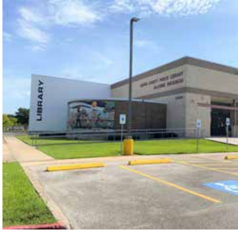
VIEW FROM NORTH EAST
