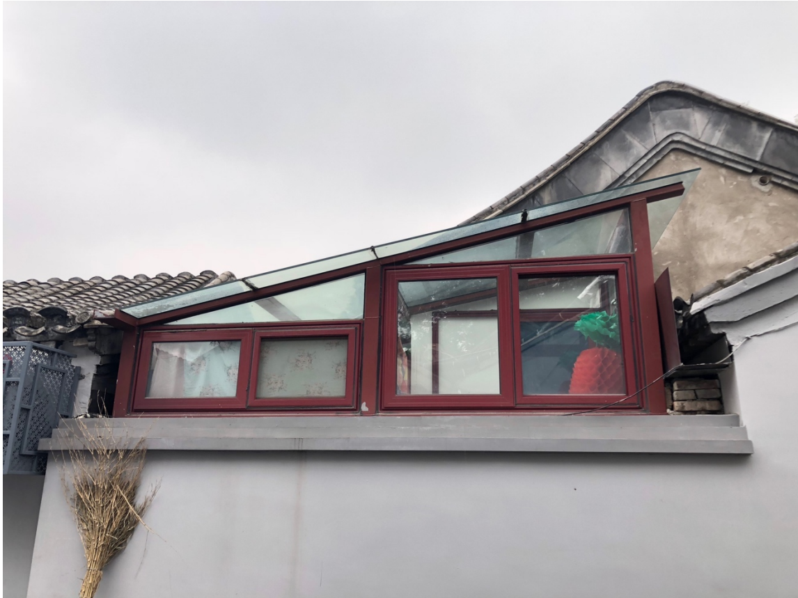
Figure 11. Residents identify constructions with non-traditional materials and appearance (such as this structure using stainless steel windows and glass ceiling) as not in harmony with the traditional characteristics of hutongs, particularly because these parts are visible on the exterior façade. Such covering structure are often built and used by the residents as climate controlled green house, shower, or storage space. Photo by the author.
