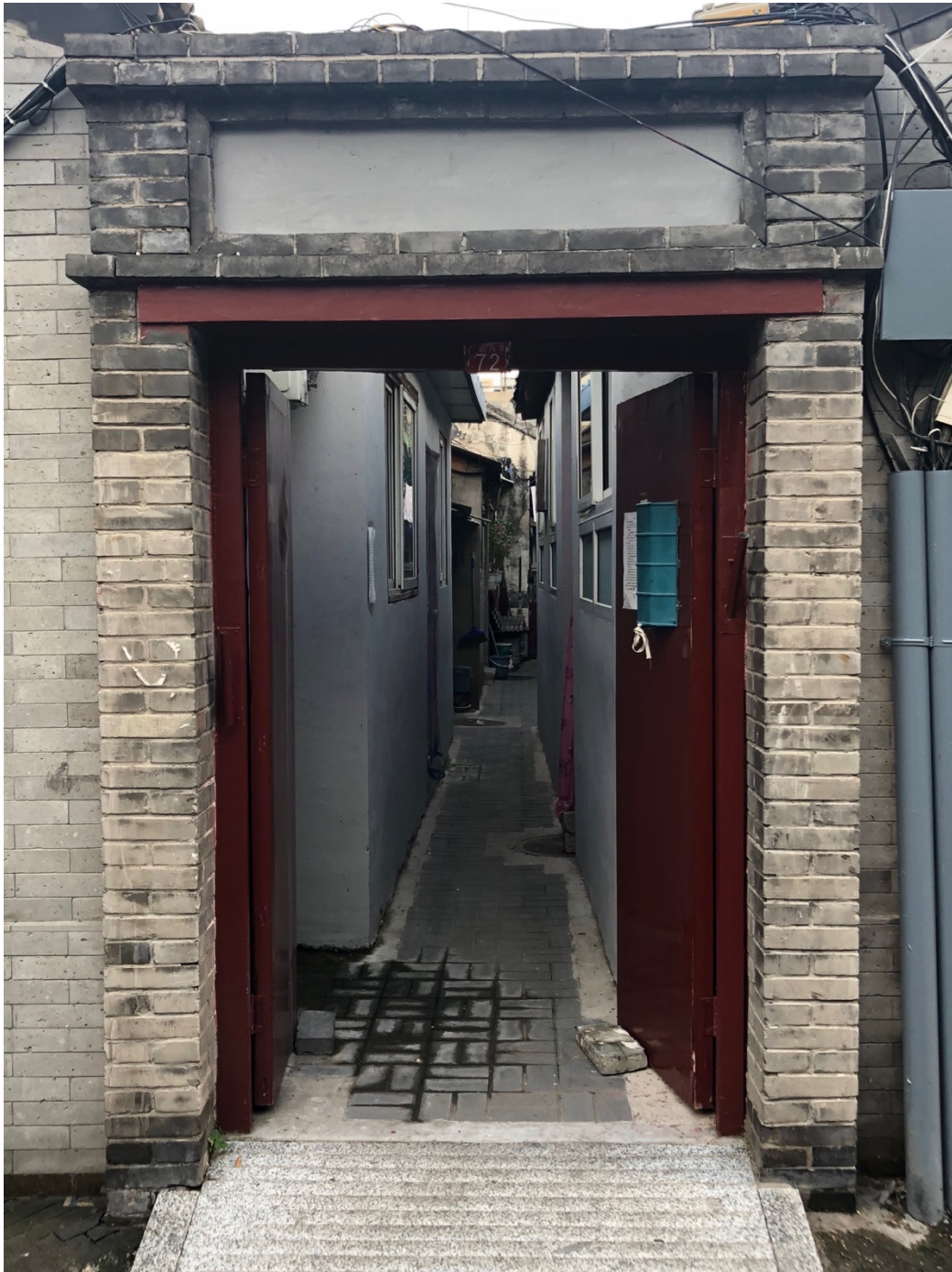
Figure 16. A typical narrow entrance way from the backdoor of a courtyard house complex. Due to the limitation of living space, “unlicensed and illegal” additions were built by many households sharing the same in-courtyard semi-public space, resulting in narrow entrance ways, which only allow one person to walk through at the same time. Photo by the author.
