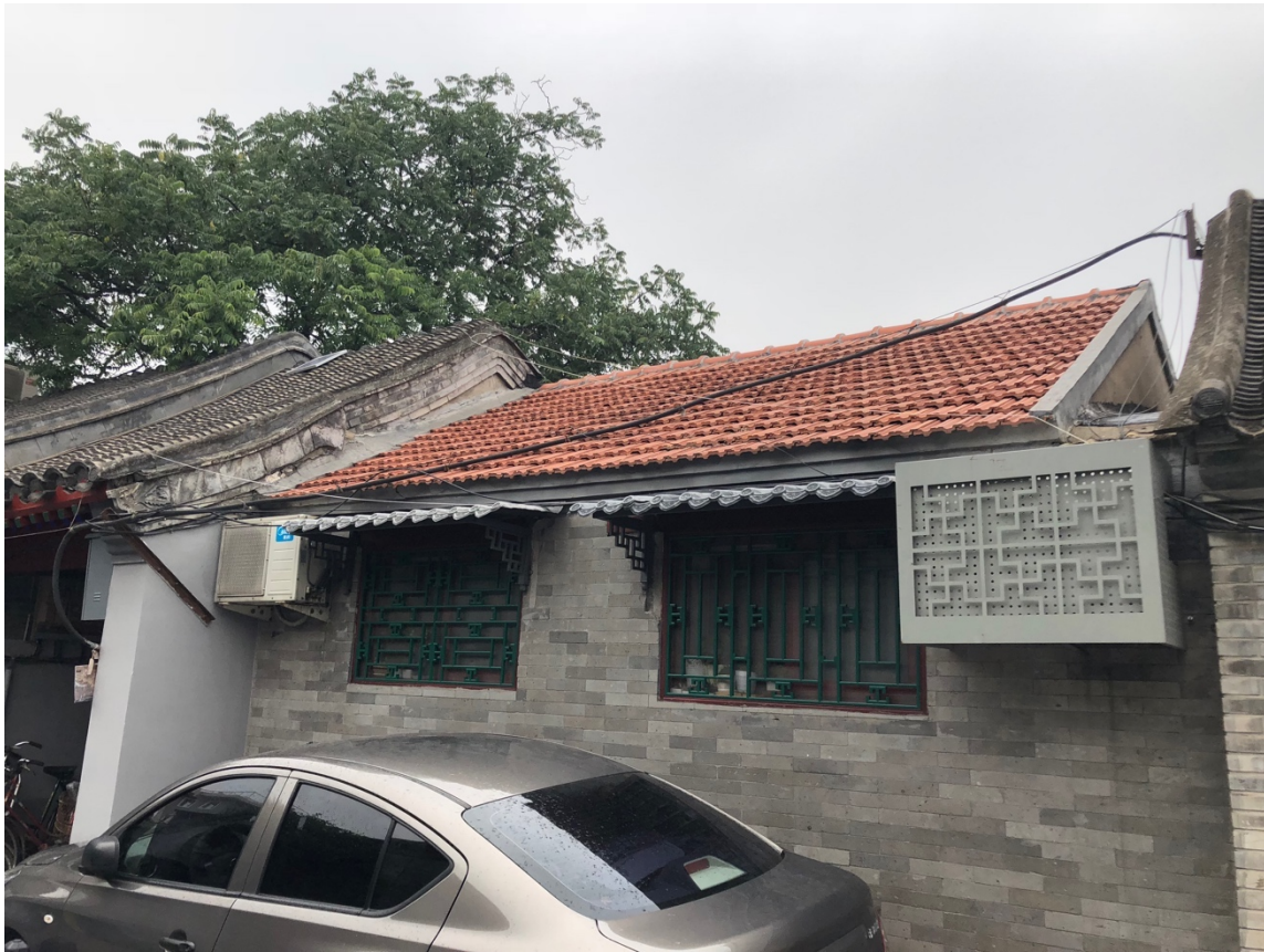
Figure 10. Red brick roof tiles used by one household. This practice (often cheaper than using grey brick roof tiles) is identified by residents as not in harmony with the traditional characteristics of hutongs, as grey brick roof tiles are the conventional material used for courtyard house roofing. Photo by the author.
