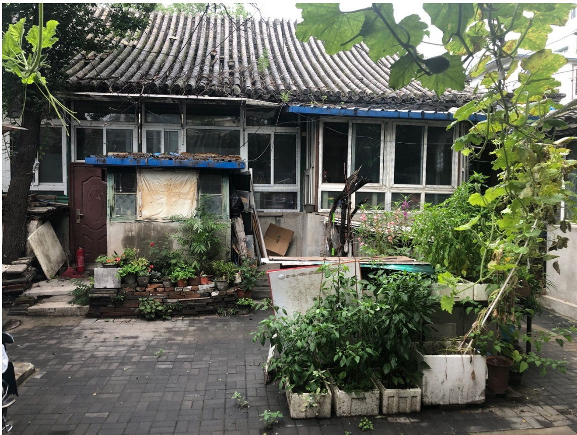
Figure 14. Typical “unlicensed and illegal” additions built inside of courtyard houses. The additions with blue flat roof are attached to, not part of, the original single-story building. Photo by the author.
