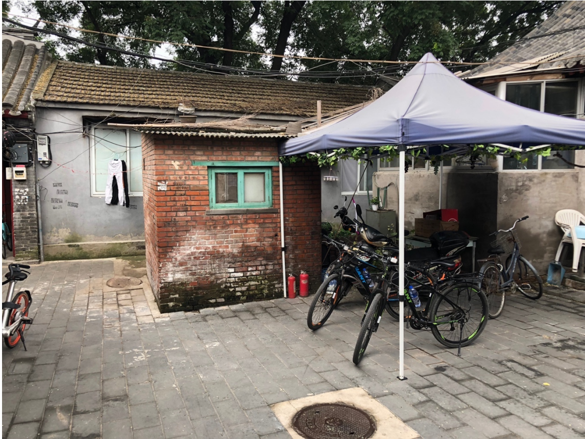
Figure 15. Typical stand alone “unlicensed and illegal” structures built inside of courtyard houses. This kind of structures are usually used as kitchen or storage room. Photo by the author.
