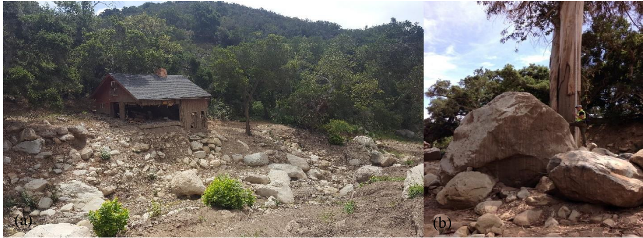
Figure 1. (a) Dwelling damaged by a 2018 Montecito debris flow along Romero Creek in Montecito, CA. (b) Boulders transported by debris flows along western Transverse Ranges with a 2 m human for scale. These flows were generated by the Thomas Fire and an intense rain event. Photograph credit: Derek Cheung, 2018.
