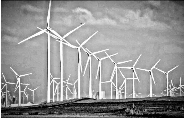
Figure 16 Wind farm in West Texas. (Photo by J. Giardino, 2019). Reprinted with permission from Aguilar et al., 2020.
