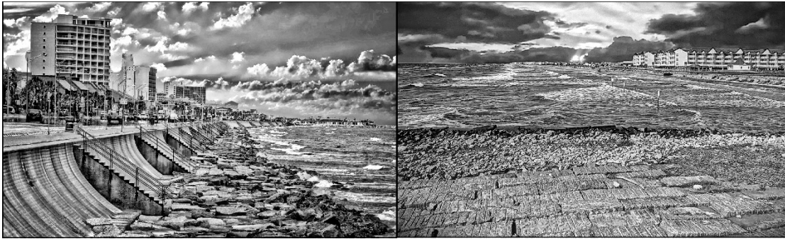
Figure 6 The seawall along Galveston Island, Texas. Note the lack of a sand beach in front of the seawall. (Photo by J. Giardino, 1988). Reprinted with permission from Aguilar et al., 2020.
