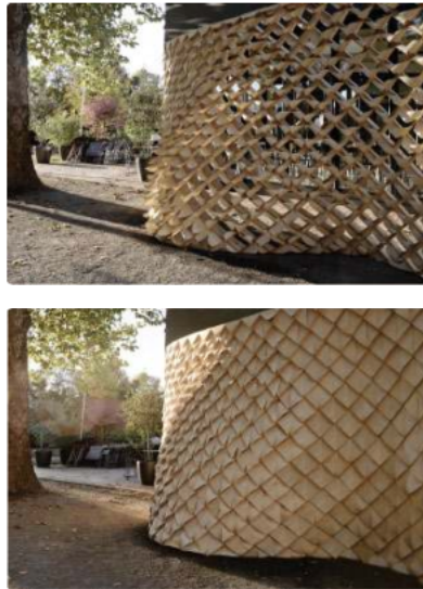
Figure 5.4: A full-scale responsive prototype of “Hygroskin” in the open (top) and closed (bottom) positions [17].
