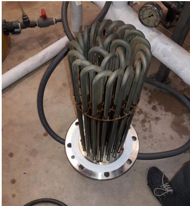
Figure 3.7. 50 kW heater prior to installation into the steam generator.
