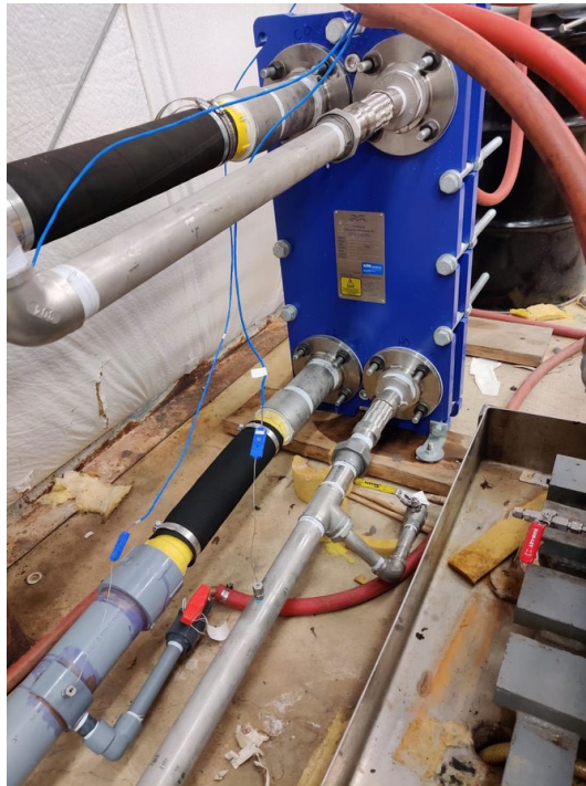
Figure 3.31. HRS piping connections to HRS heat exchanger.
