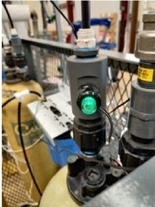
Figure 3.1. Culligan® water filtration system indicator light. Turns red when the tank needs to be replaced.
