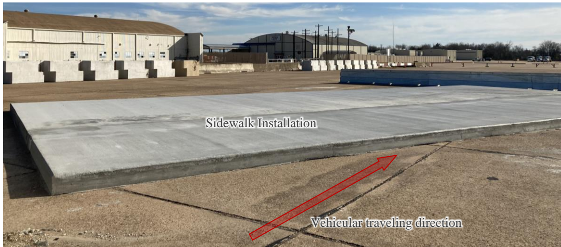
Figure 3.1 Installation of a sidewalk with a curb
