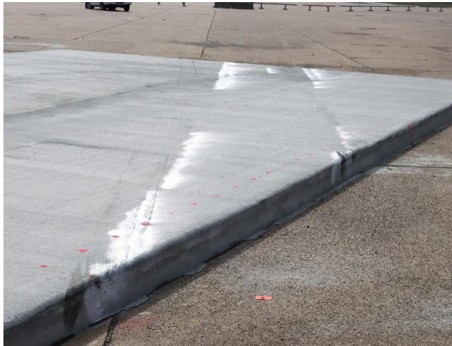
Figure 3.16 Tire traces on the sidewalk after the test completion
