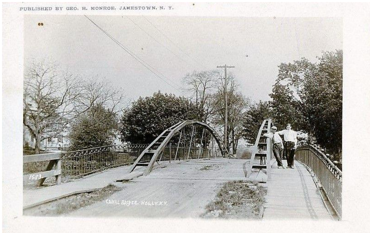
Figure 16. A 75-Foot Whipple Bowstring Arch Truss Bridge with Pedestrian Sidewalks.
