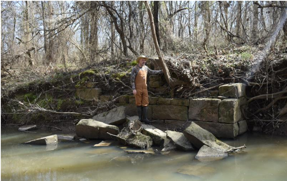
Figure 10. Eastern Masonry Stone Abutment at Redbank Creek. (Kyle Burch, February 2020)
