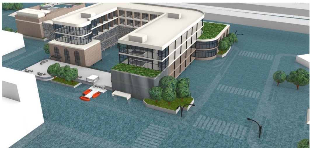
Figure A.21: The Refuge Hotel – site during flood conditions (secondary function as surge facility)
