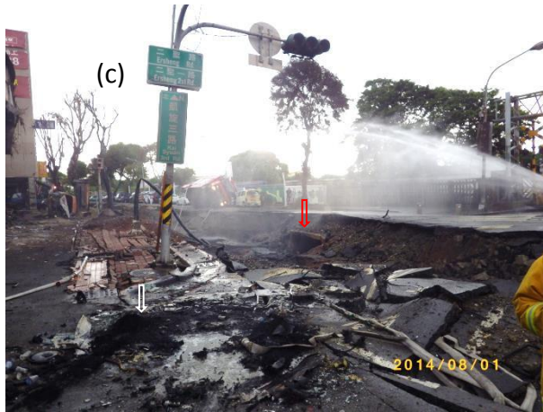
Figure 4: Photos of the fire after the explosion on the north side of junction of Kaixuan 3 rd road and Ersheng 1 st road. Time of the photos: (a) 12:00 am (b) 06:00 am (c) 07:05 am. Red arrow indicates the location of storm water trench branch with the leaked pipeline. Yellow arrow indicates the fire truck engine suspected to be the ignition source. White arrow indicates the char from burnt fire truck tire. Note for the road sign in front of the engine remained intact.
