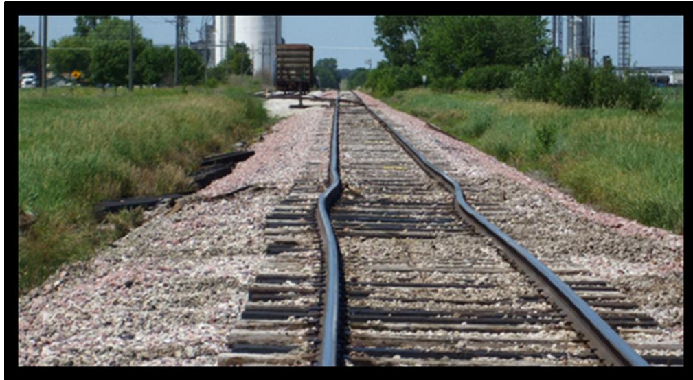
Figure 1 Photograph Showing Thermally Induced Buckling of a Railway (Reprinted with Permission from Allen and Fry, 2017)
