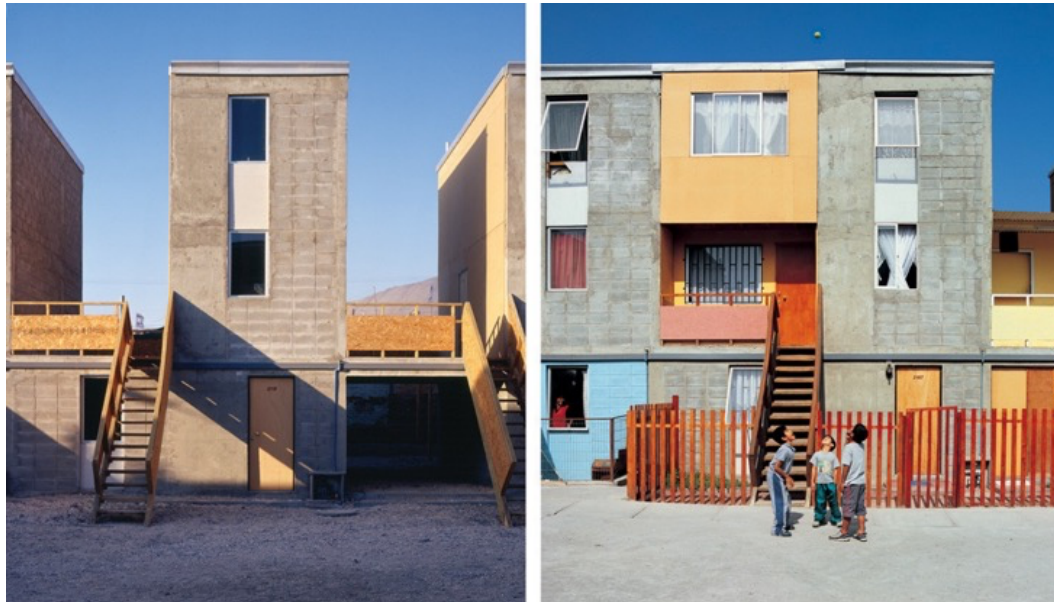
Figure 63: Before and after showing the result of user's appropriation of the design. Quinta Monroy (2003) by Alejandro Aravena. Reprinted from Aravena & Iacobelli (2012)
