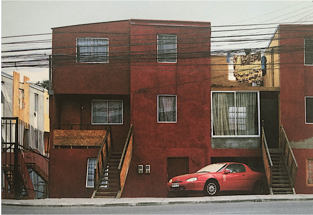
Figure 67: A finished house from a residents' perspective. Quinta Monroy (2003) by Alejandro Aravena. Reprinted from Aravena & Iacobelli (2012)
