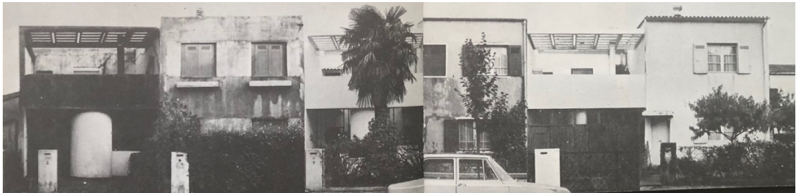
Figure 38: Exterior design alterations at Pessac (1926), by Le Corbusier. Reprinted from Boudon (1979)
