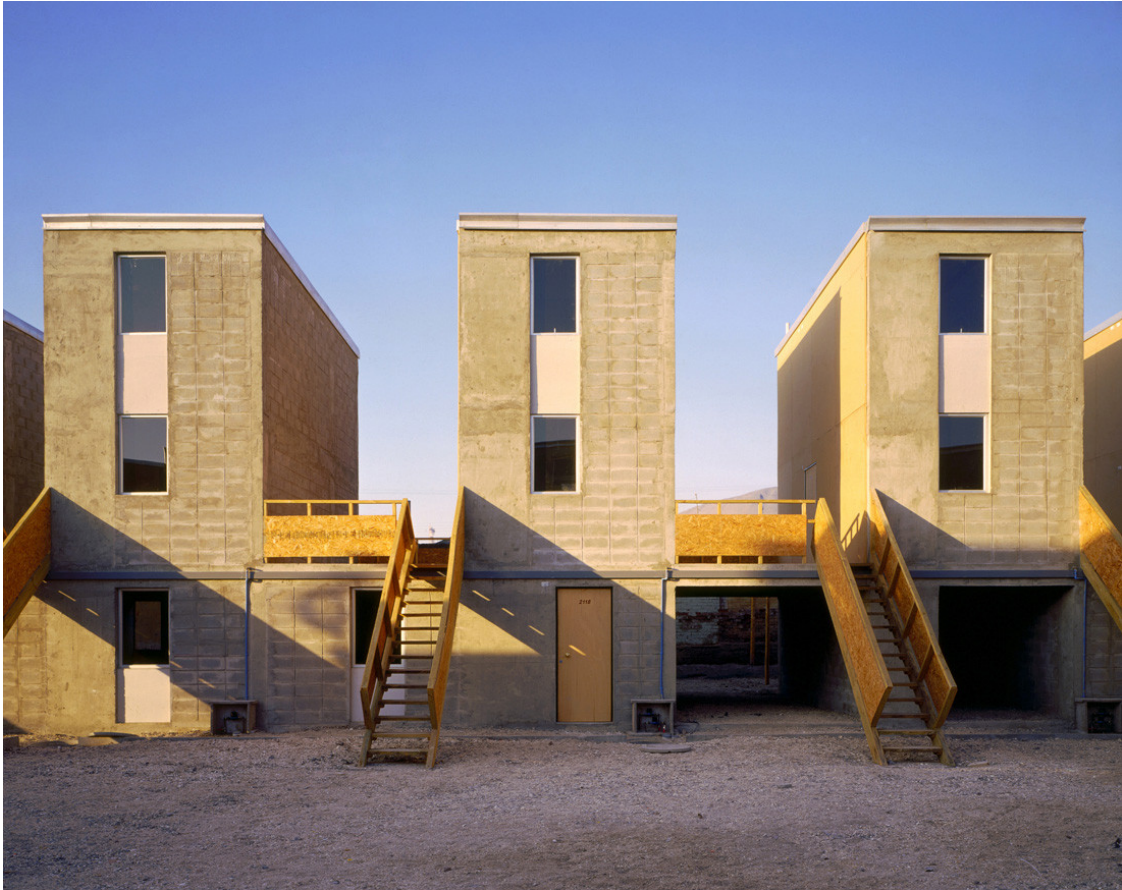
Figure 66: Unfinished project from the architects' perspective. Quinta Monroy (2003) by Alejandro Aravena. Reprinted from Aravena & Iacobelli (2012)
