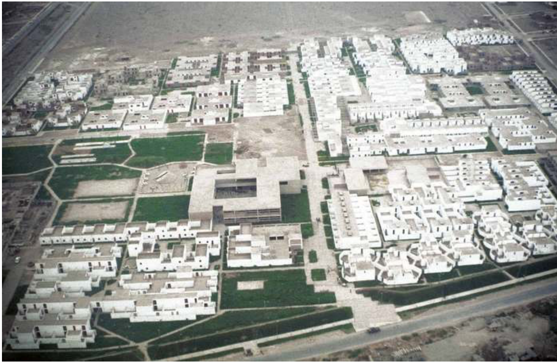
Figure 3: Site plan of PREVI (1969), showing housing organization. Image from Col·legi D'Arquitectes de Catalunya at http://quaderns.coac.net/en/2013/05/previ-lima/
