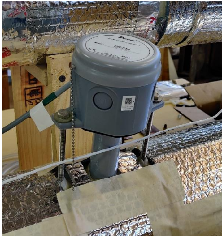
Figure 7 CO 2 and RH sensor
