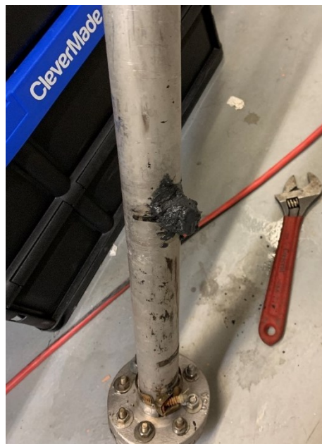
Figure 19: Leak test of point B
