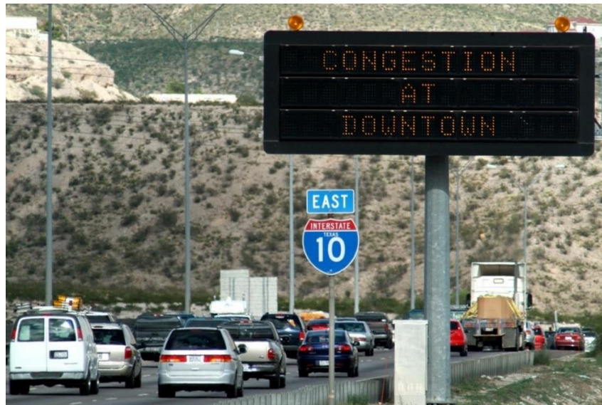
Figure 7. Use of ITS devices for controlling traffic during the peak hour period (Photo courtesy of Texas A&M Transportation Institute)
