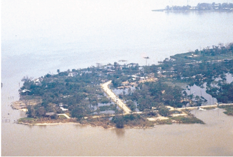
Figure 10: Hurricane Alicia (1983) destruction of Scott Bay, Brownwood neighborhood (White et al., 2003). Picture from Harris-Galveston Coastal Subsidence District
