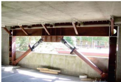
c) Retrofit with fluid viscous dampers
