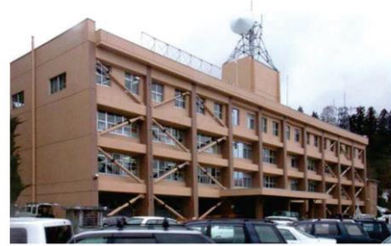
b) External retrofit of a building
